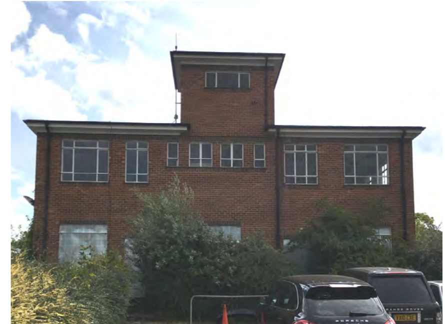
Figure 17: Dis-used building to centre-east of Site
