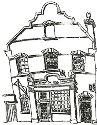
2. Hampton Hill Dairy at 55 High Street
