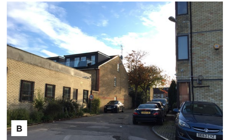
Neighbouring buildings façades are of minimal interaction
