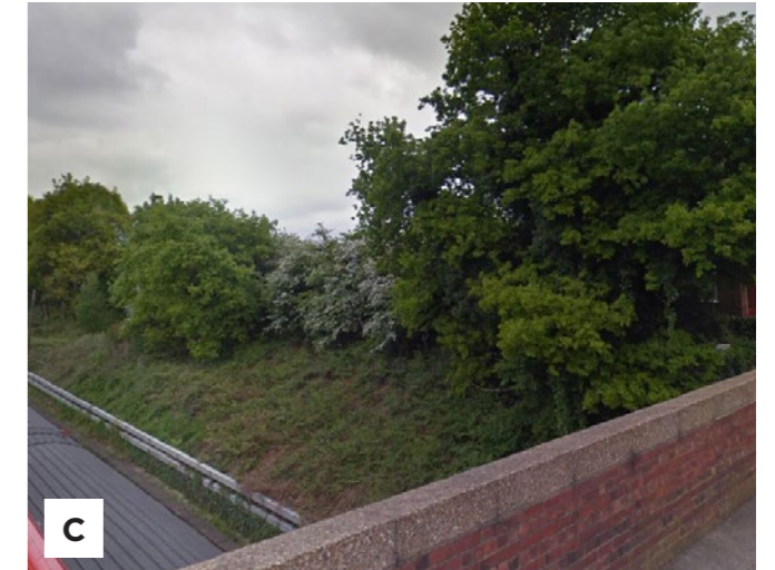
C Railway bank of dense shrub and tree vegetation
