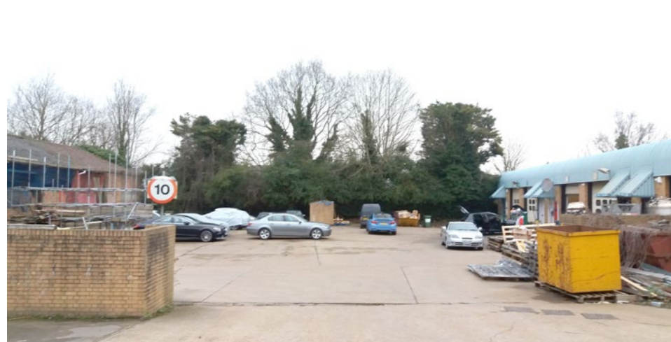
7. View west towards railway, with Units 2-6 to the right and Atcost Structure to the left
