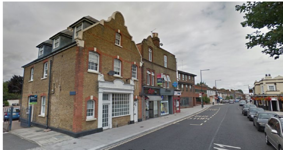
4. Buildings 53 at High Street
