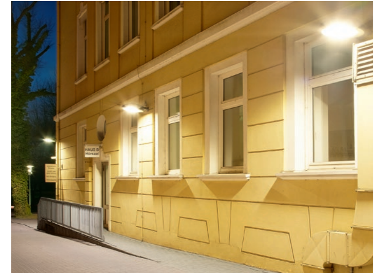
Examples of bracket mounted lighting unit
