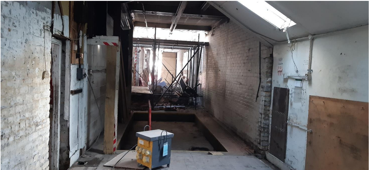
Former vehicle ramp pit
