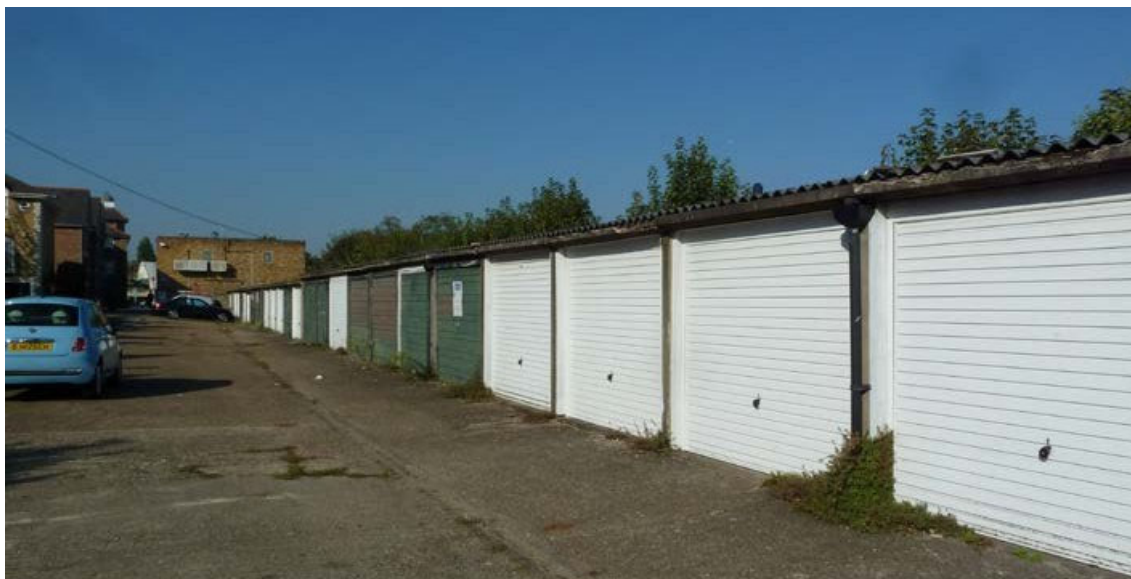
View of site looking west on South Worple Way
