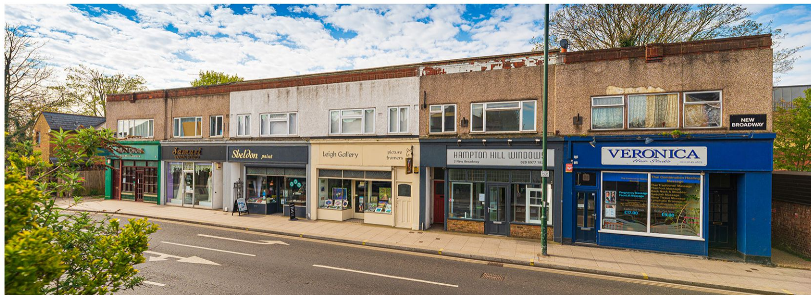
FIGURE 04 - EXISTING 1-6 NEW BROADWAY (NO. 3&4 IN MIDDLE)
