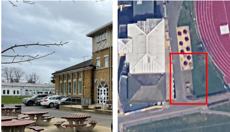
Photos of the existing east facing elevation
