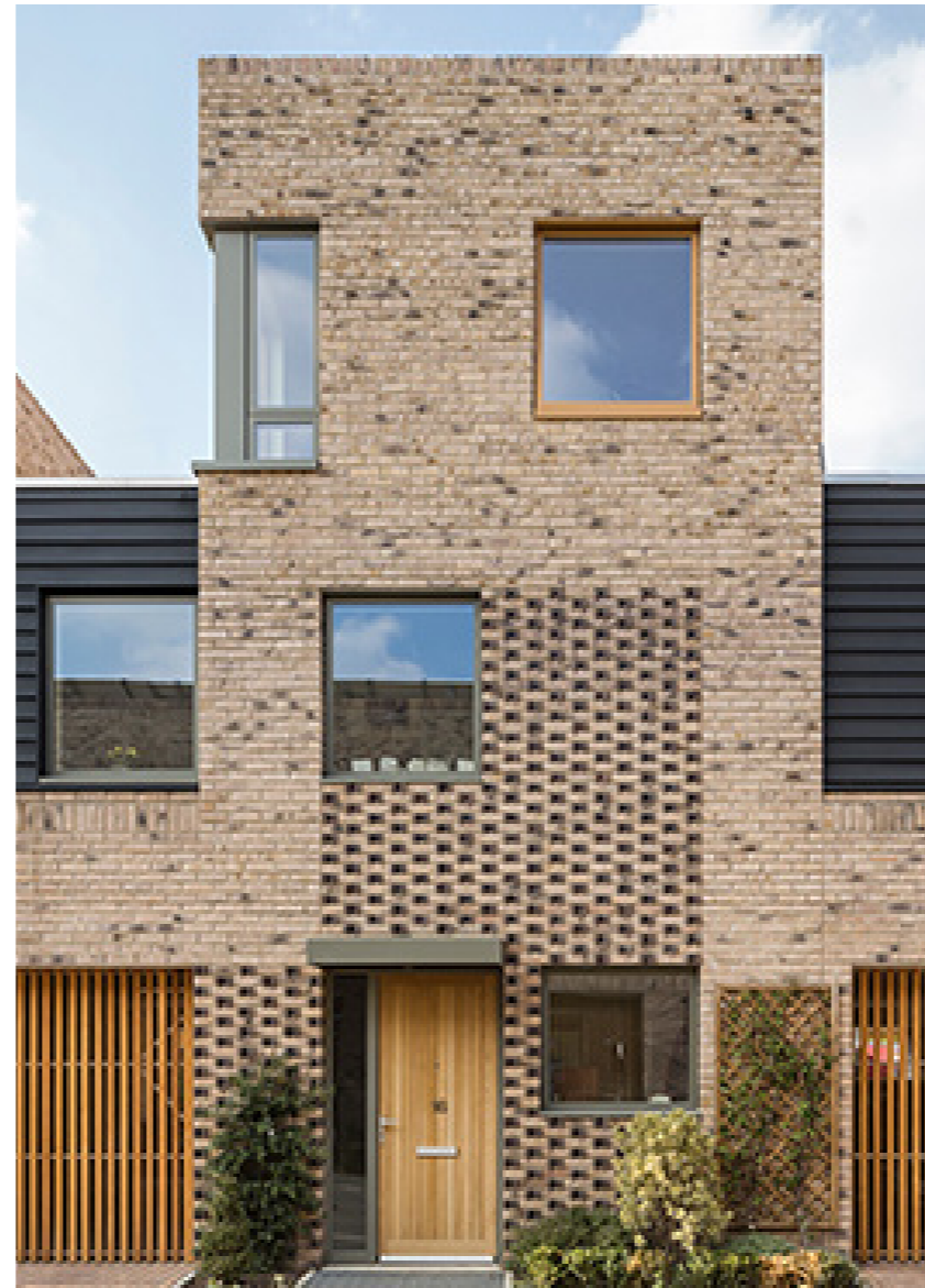
Example of timbers secondary elements only
