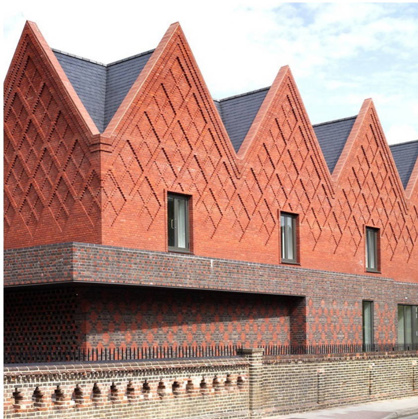
Example of contemporary detailing of vernacular form
