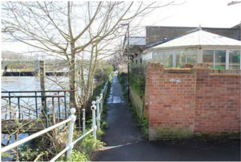
Existing photo of the Boathouse and river walk showing the narrow footpath and overhang from the building
