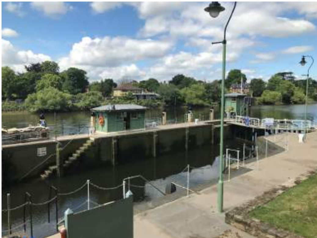
Figure 16: View of the Site from the northeast (opposite bank Thames towpath) with Richmond Lock and its variety of kiosks in the foreground
