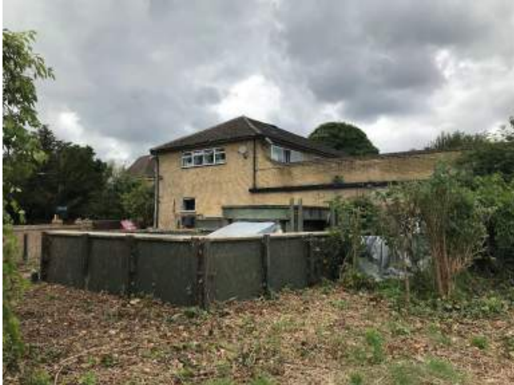
Figure 12: View of the Boathouse and associated air conditioning external plant from the southeast
