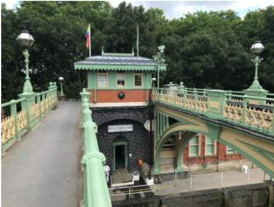
Figure 19: Former toll booth with fretted timber canopy at upper level to the Surrey side (east) side of the footbridge
