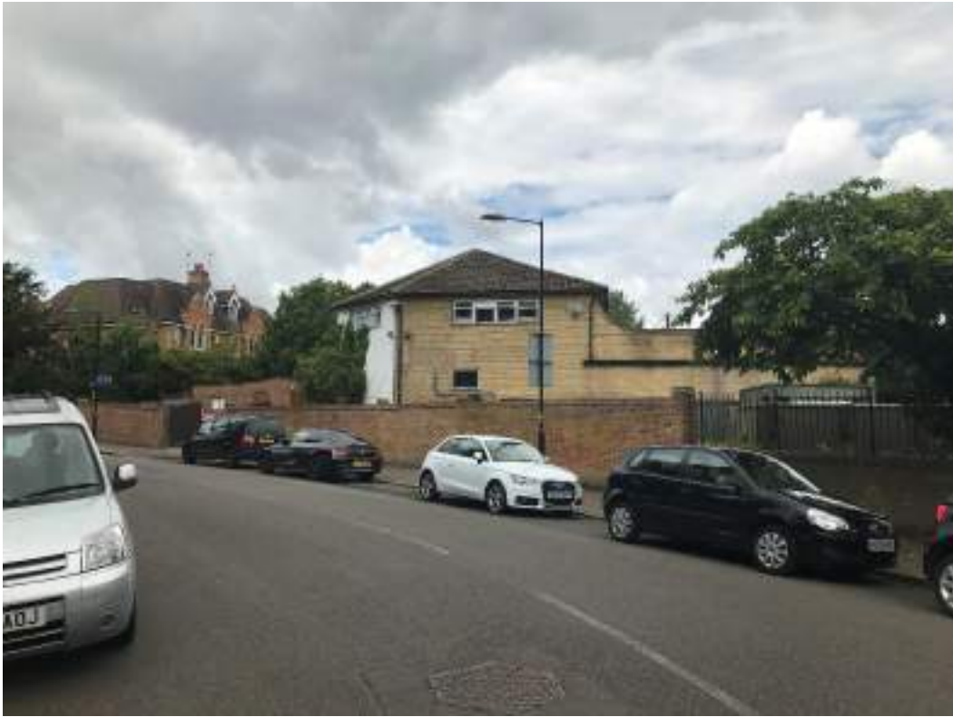
Figure 13: View of the Site from Ranelagh Drive to the south
