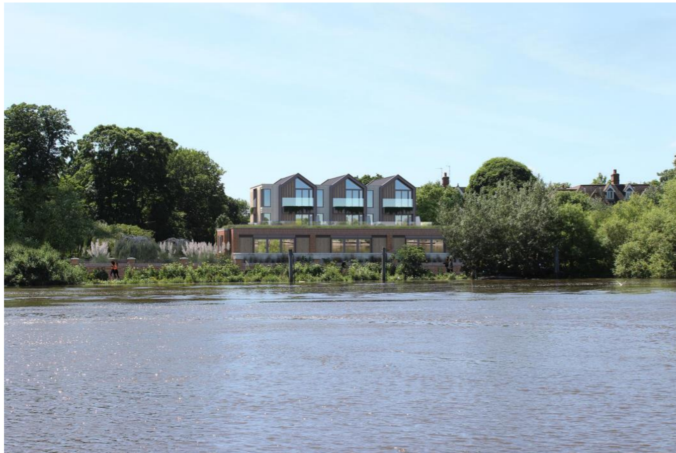
South view of The Boathouse
