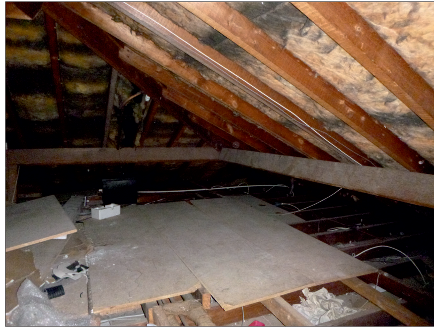
Photograph 2: Showing the well-sealed roof space.
