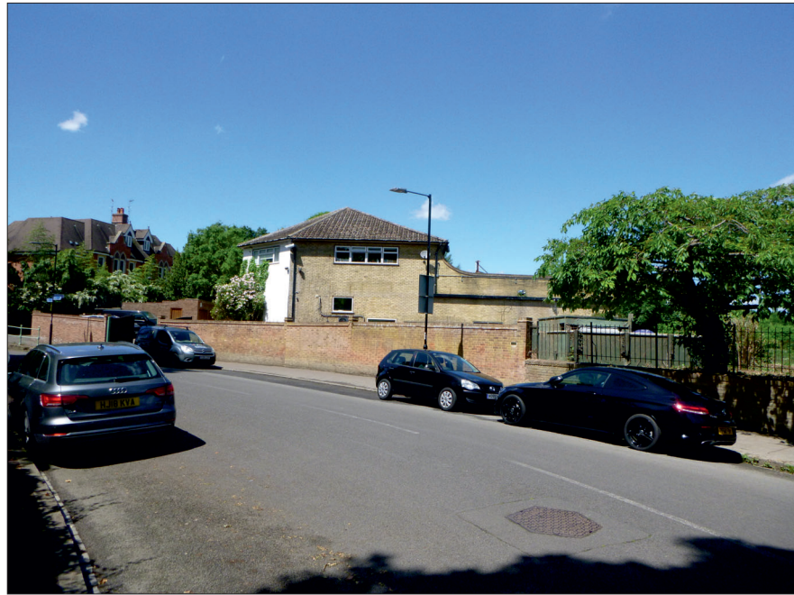
Photograph 1: Showing the site and the building 'The Boathouse'.
