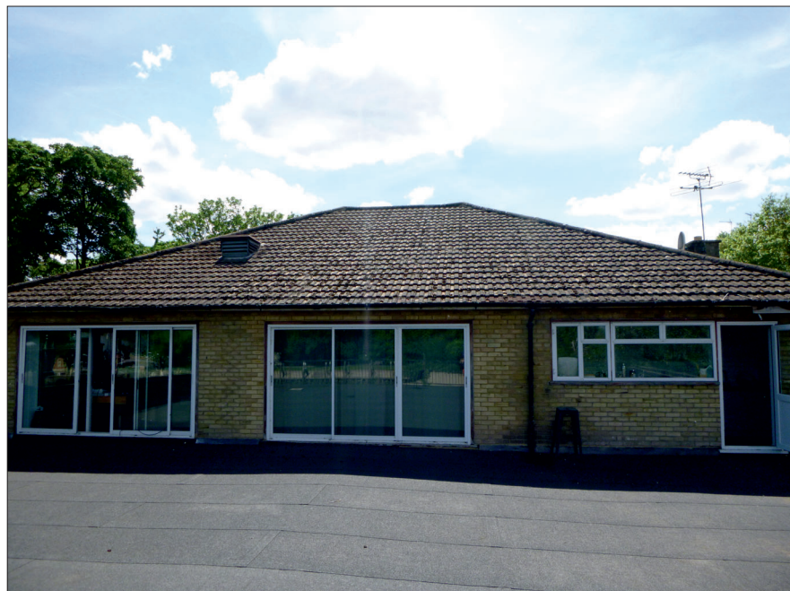
Photograph 3: Showing the well-sealed tiled roof.
