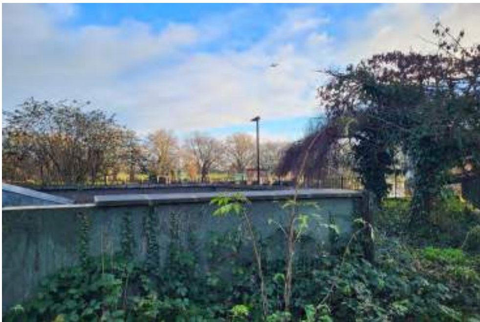
General Site View—Extractor fan enclosure
