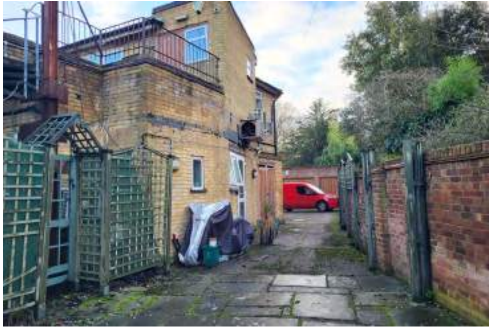
General Site View—Looking southwest
