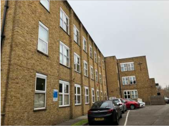
View of West Elevation
