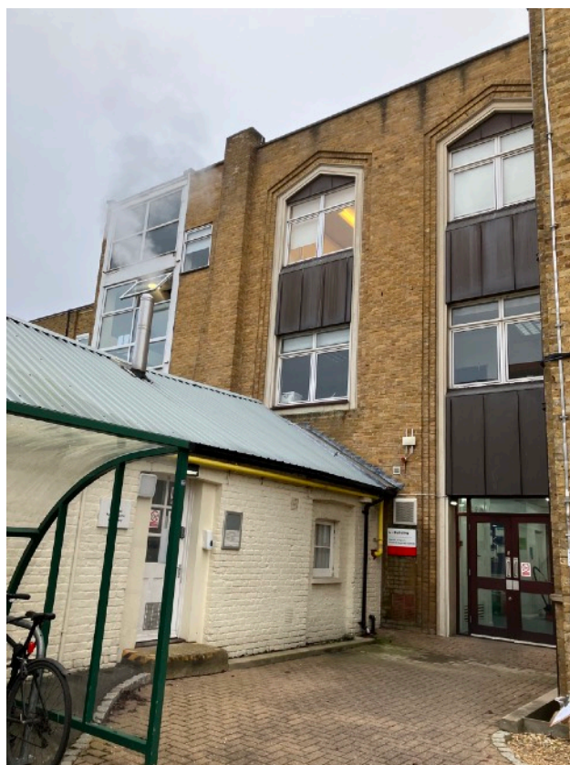
View of Block L East Elevation
