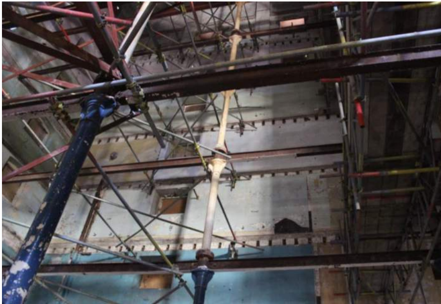
Plate 14: Interior of Maltings building, showing cast iron columns and iron I-beams (2017)
