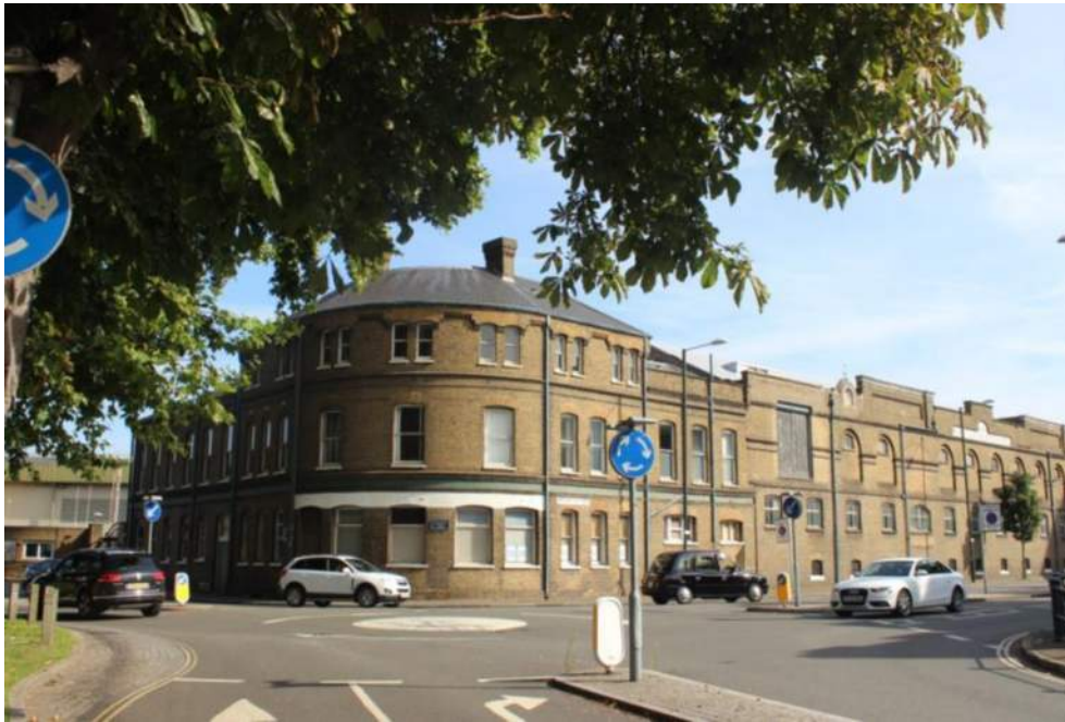
Plate 1: External, bowed, elevation of Former Hotel, facing onto the roundabout (2017)
