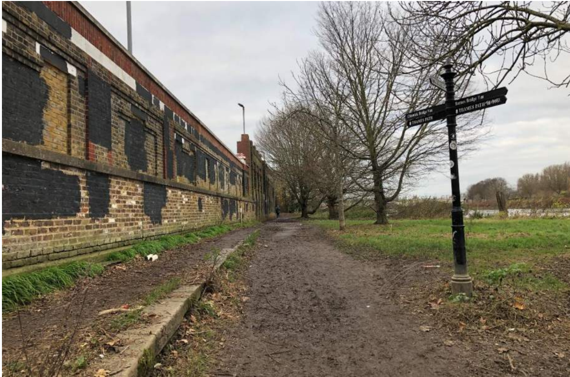
Plate 22 Sections 6 and 7 of the northern wall (2021)
