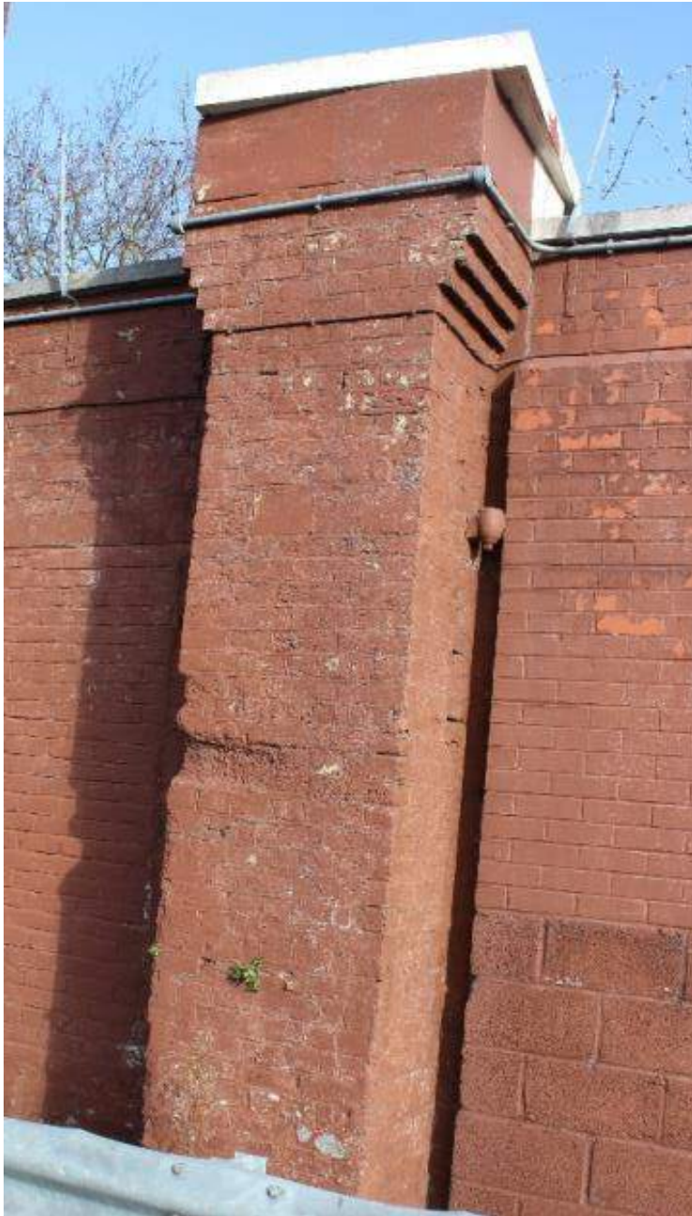
Plate 21 Interior elevation, showing gate pier and surviving hinge socket (2017)
