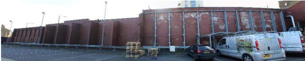
Plate 29 Internal elevation of south boundary wall (2017)
