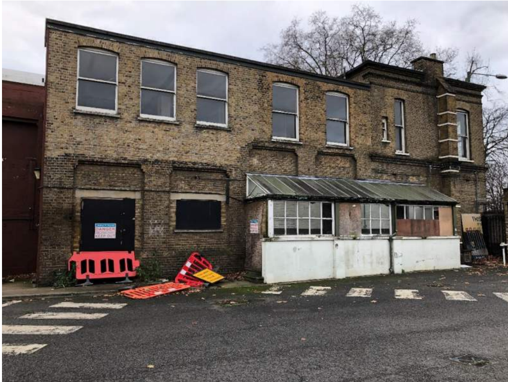
Plate 3: North facing elevation of Former Hotel (2021)
