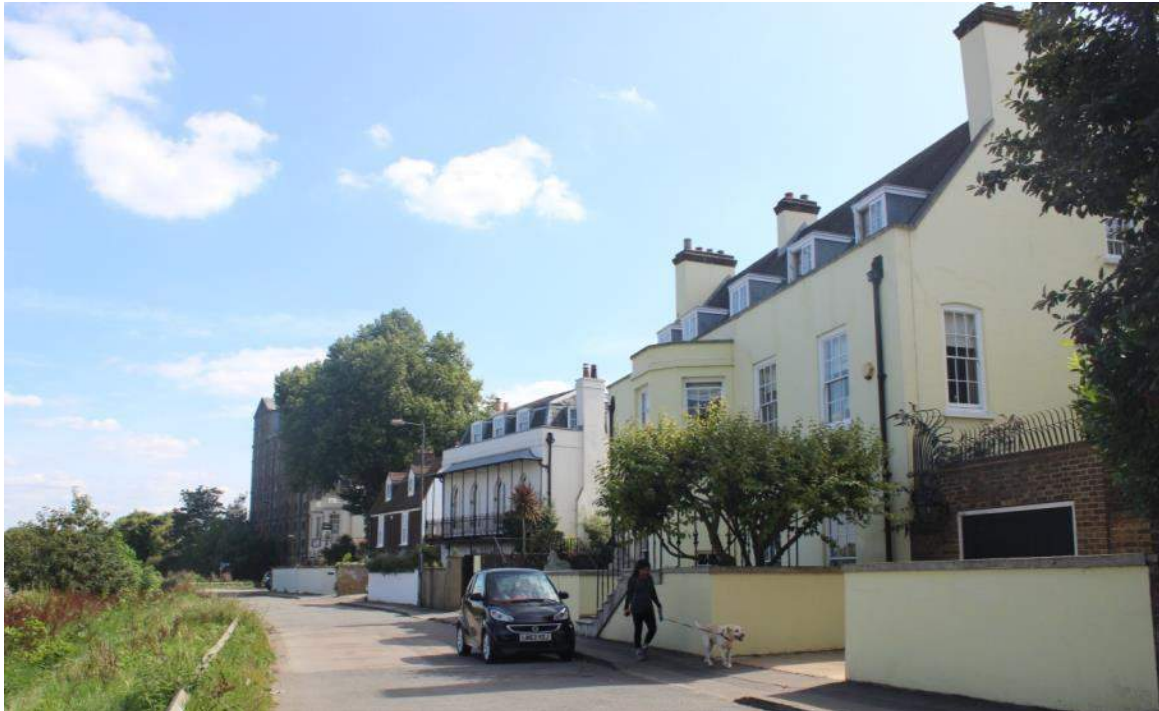
Plate 38: Grade II Listed Tudor Lodge, Thames Bank House and Leyden House (2017)
