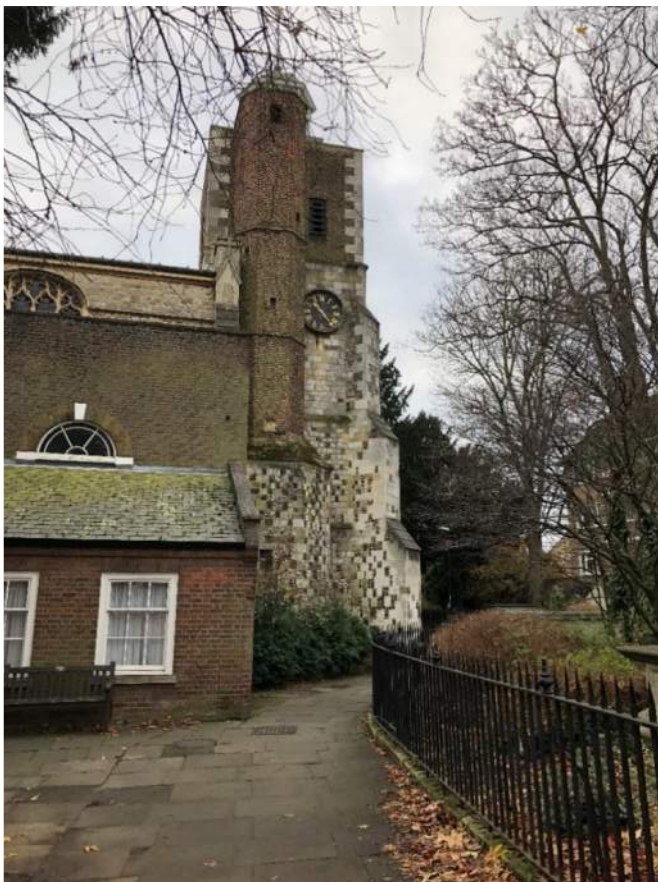
Plate 48: Grade II* Listed Building Church of St Mary (2021)
