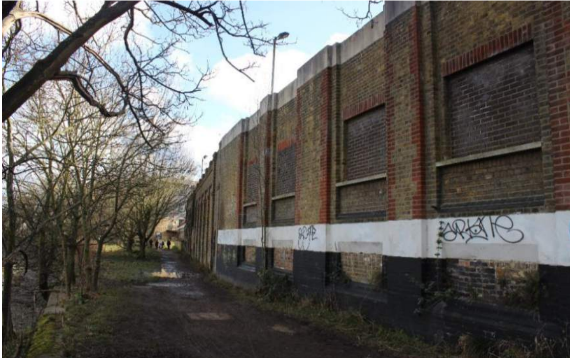
Plate 18: Section 3 - Wall of 1937 Tun Block
