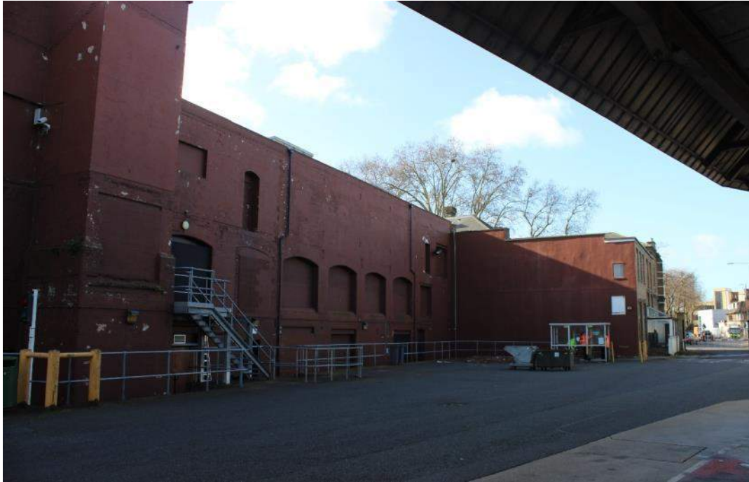
Plate 6 Northern, internal elevation of the former Bottling building (2017)
