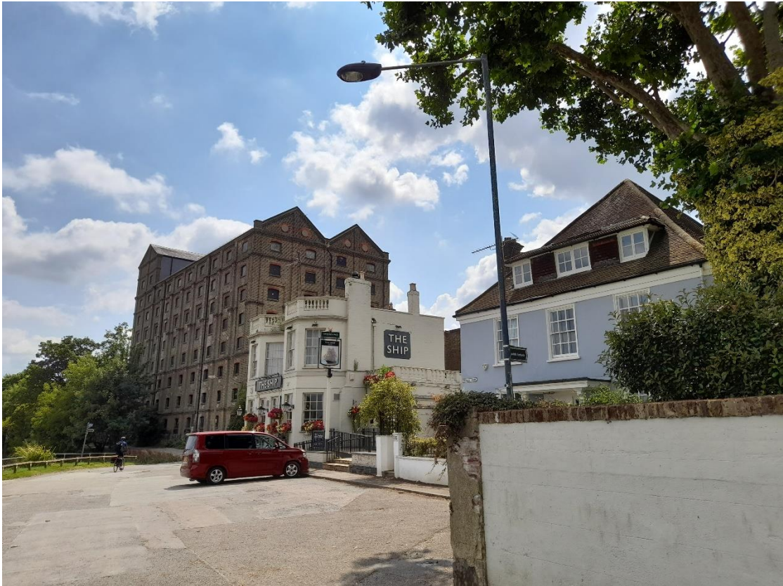
Plate 9: View towards the maltings building from the Thames Path. Existing view to south-east
