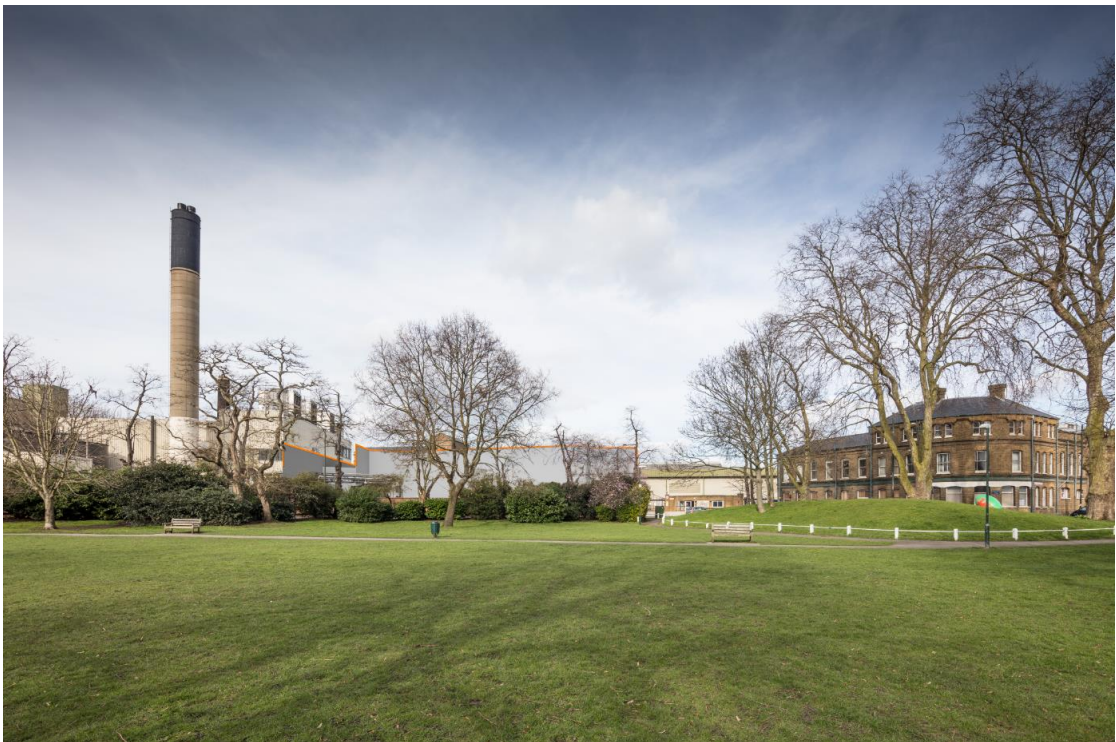
Plate 8: Photomontage of the proposed development viewed from Mortlake Green. Proposed view to north. Refer to Appendix 3 for high-resolution image
