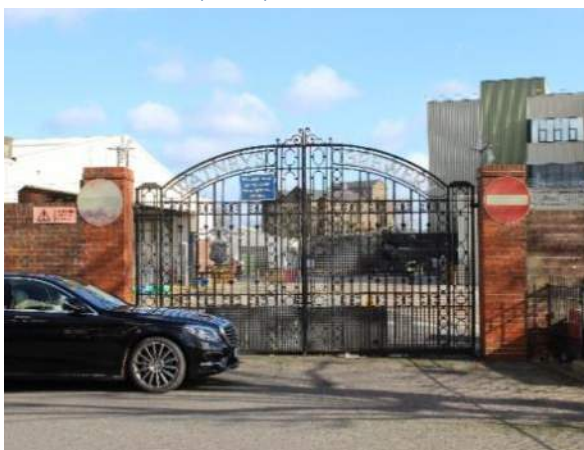
Plate 35: Gates Installed in West Site Boundary Wall (2017)
