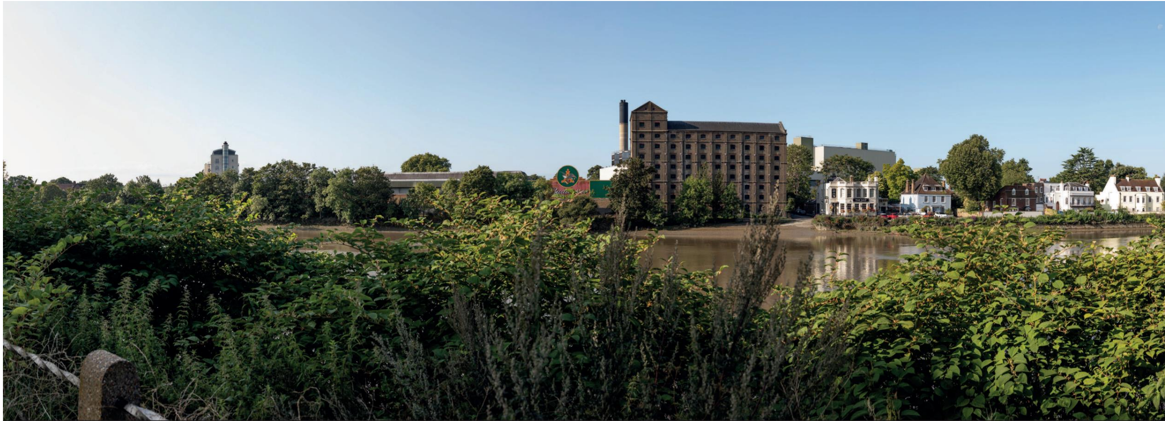
Figure 3: View towards the maltings building from Duke's Meadows. Existing view to south
