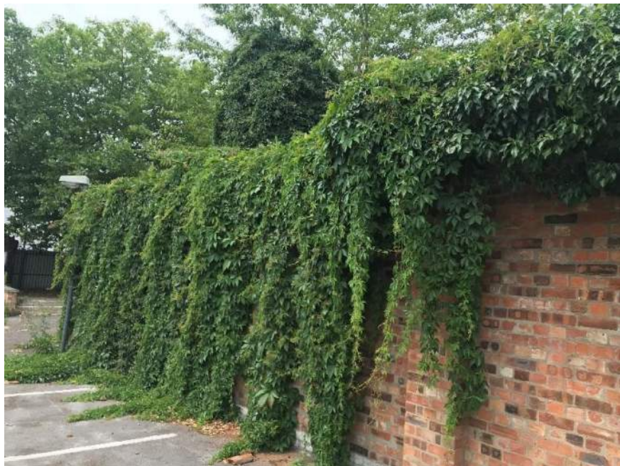
Plate 6 – Example of Virginia creeper overgrowing wall from neighbouring property within the north of the Site.
