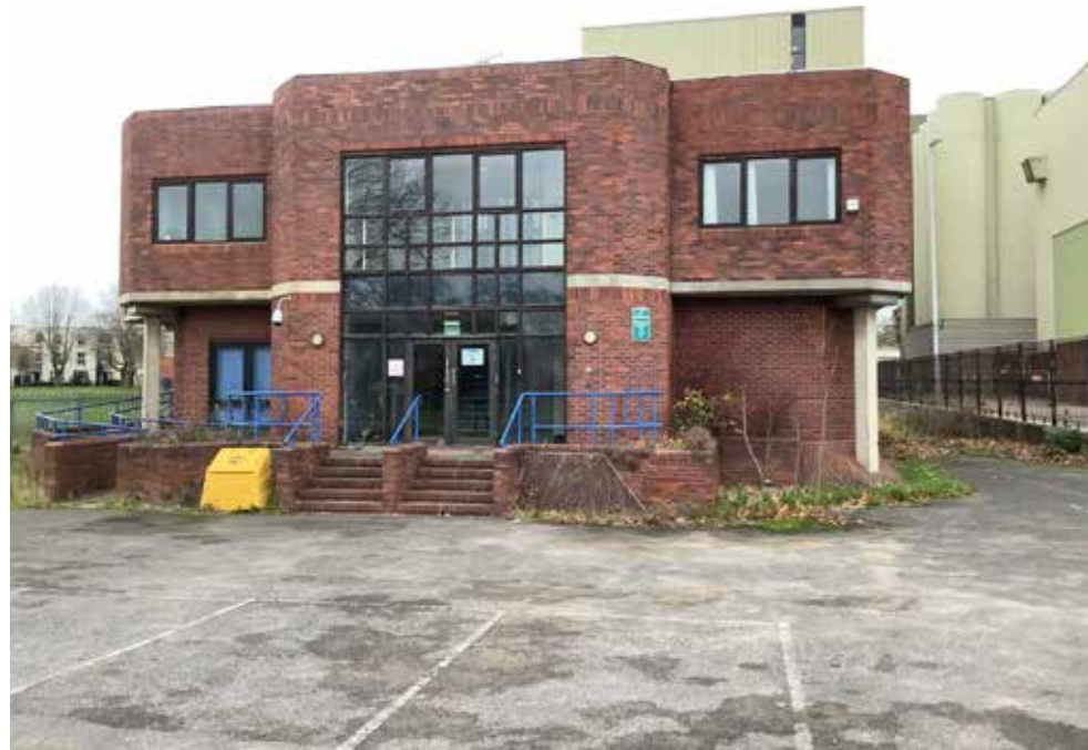
Clubhouse building at brewery West Site
