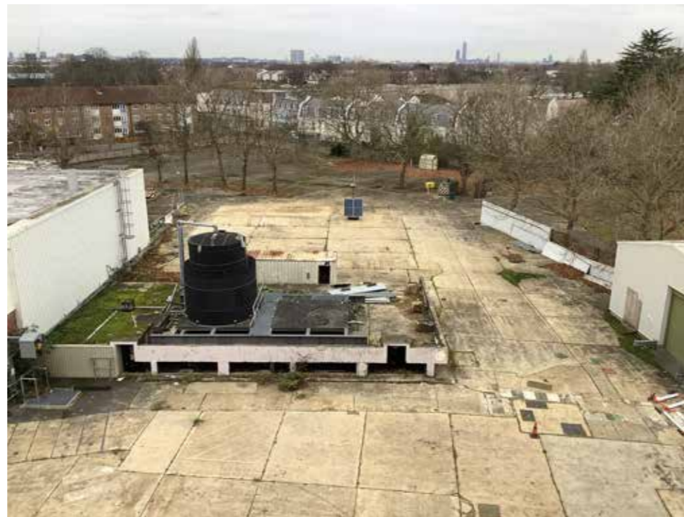
Former effluent tank and adjacent tank base at brewery West Site
