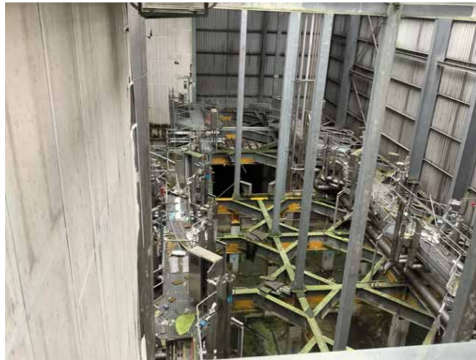
Remains of former brewing tanks, tanks removed and building partially demolished
