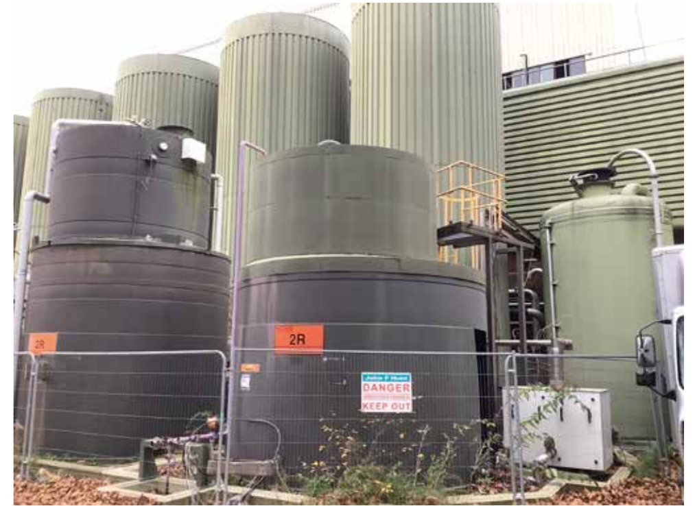
Remaining decommissioned water and chemical tanks east of brewery buildings at west site
