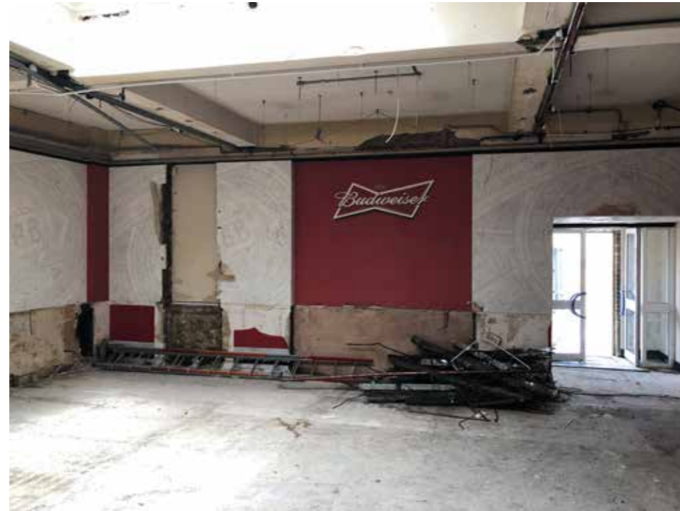
Stripout completed at eastern area canteen building
