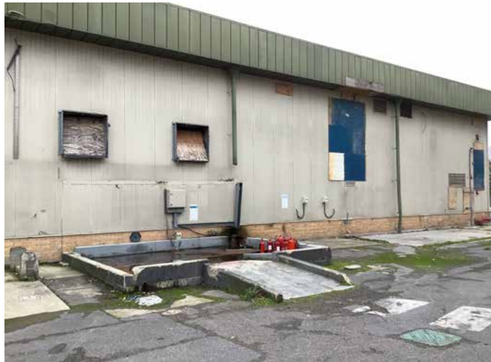
Bund for former oil tank at East Site bottling building, now removed from Site
