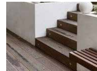
Steps responding to levels change with associated handrails
