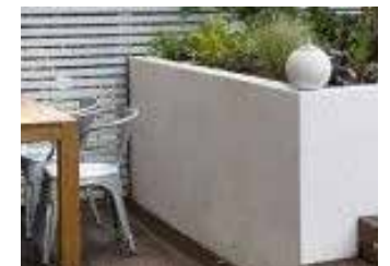
Retaining wall for level change
