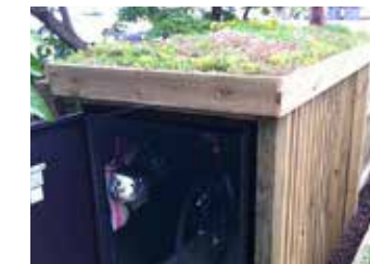
Cycle store with green roof
