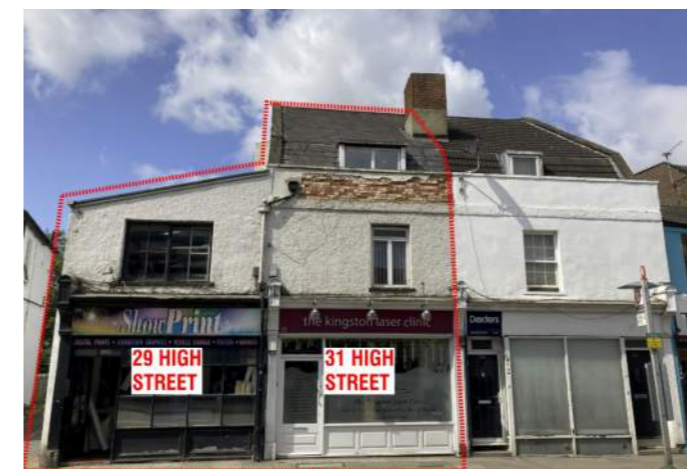
Figure 2.3 Existing Building Facade
