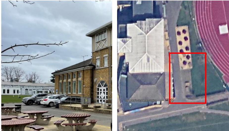
Photos of the existing east facing elevation
