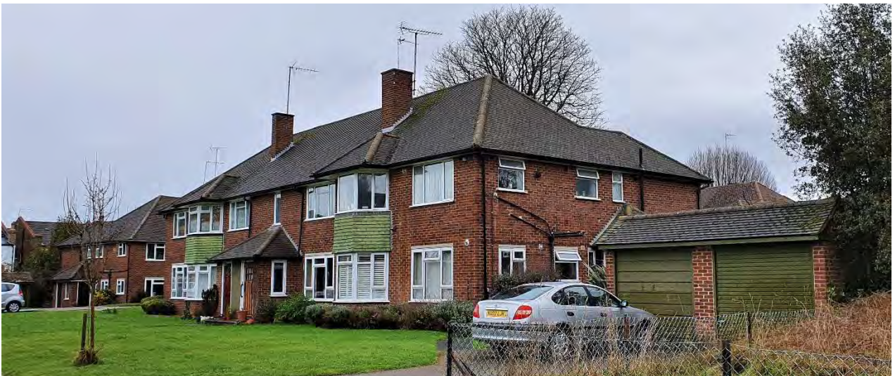
Fig.5 A typical 6-unit maisonette block and twin garage unit north of the site on Roseleigh Close
