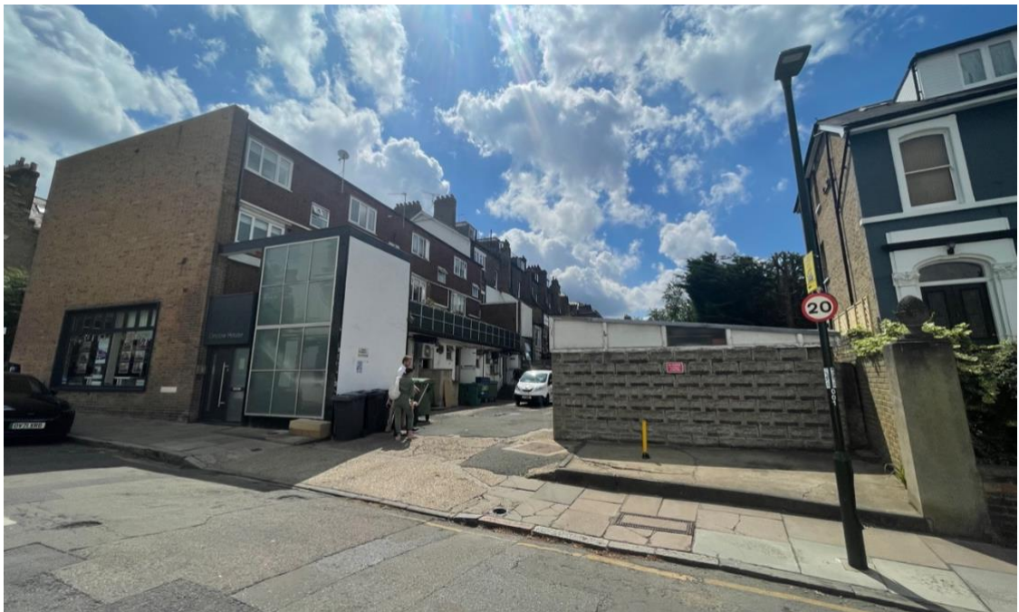
Fig. 10: Looking into the Site from Onslow Road. The visual and aesthetic disconnect between 19 – 23 Friars Stile Road, the rear stair core, hard standing and garages is very apparent in this particular view.
