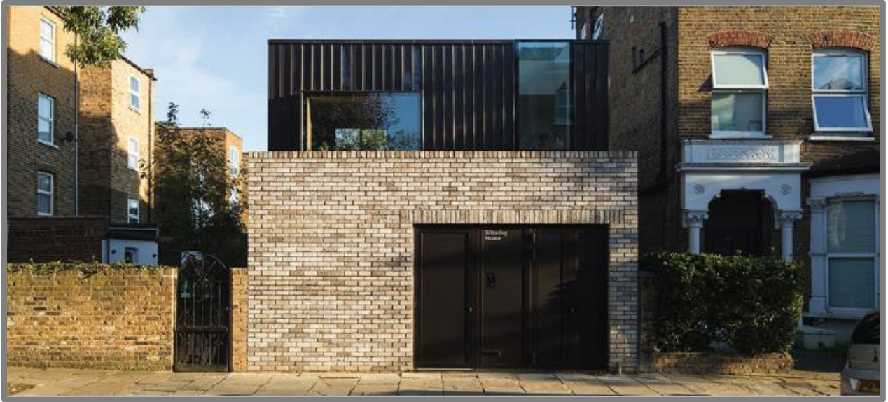
Figure 8 - Wittering House - High quality contemporary infill in Hackney
