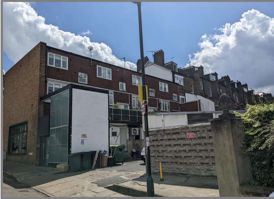
Figure 6 - Application site from Onslow Road
