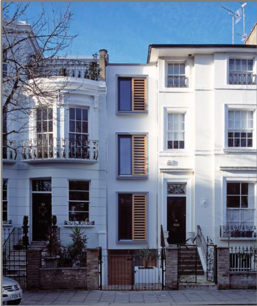
Figure 11 - Gap House, Bayswater
