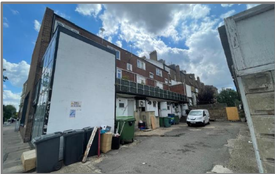
Figure 7 - Application site from Onslow Road
