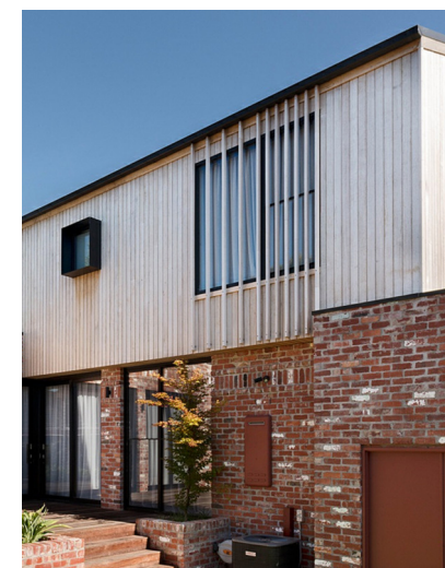
Timber fins over windows
