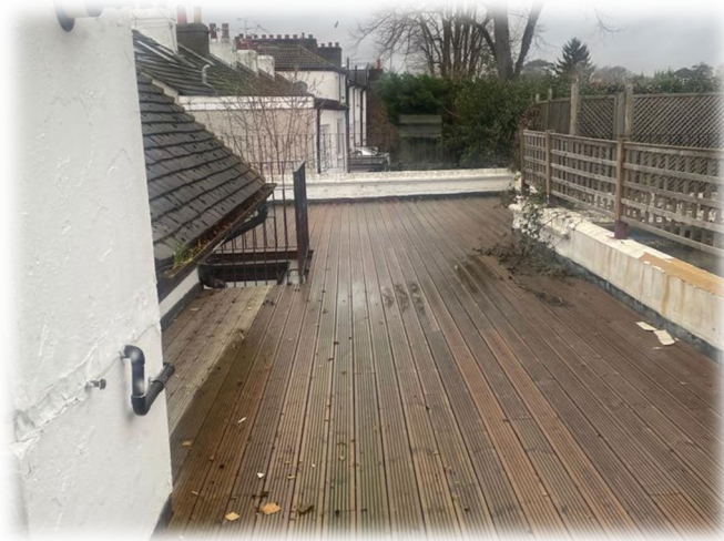
REAR TERRACE ACCESS IMAGE
