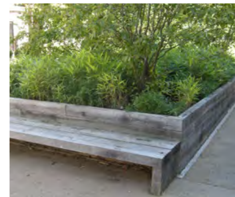
Raised podium planters
