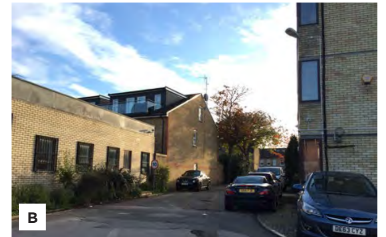
Neighbouring buildings façades are of minimal interaction
