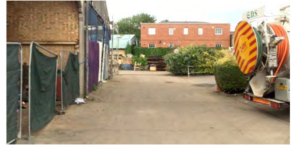
3. View north from the central zone, with Atcost Structure to the left
