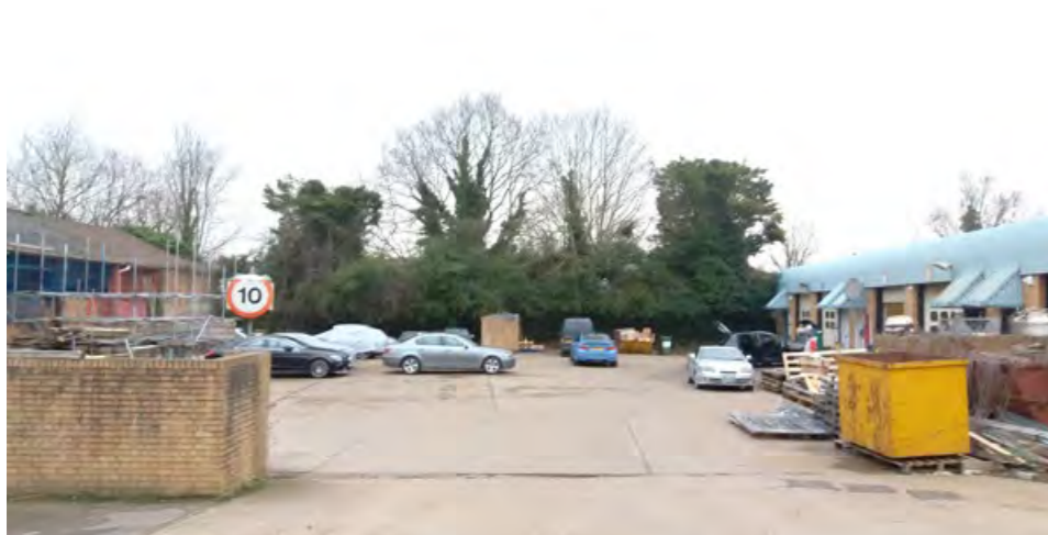
7. View west towards railway, with Units 2-6 to the right and Atcost Structure to the left
