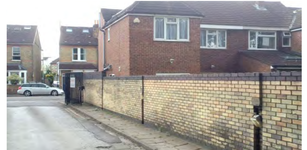
6. Access road view looking south on to Holly Road, rear gardens of Holly Road houses visible
