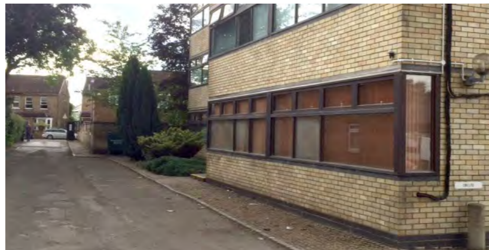
8. Access road view looking south on to Holly Road, St Clare House to the right and substation access behind it
