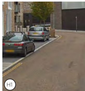
H1 Asphalt carriageway with exposed natural aggregate
