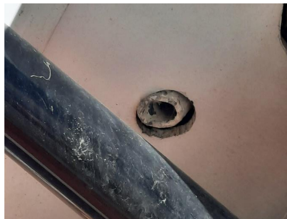
Plate 4.23: Pipe Hole (Southern Aspect)
