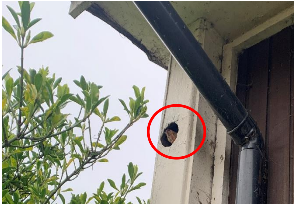
Plate 4.21: Pipe Hole (Northern Aspect)
