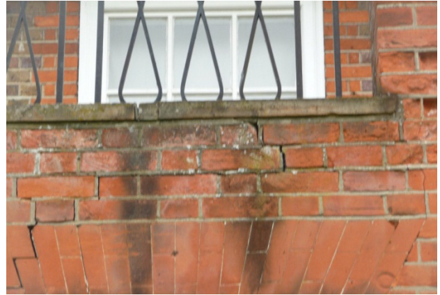
Cracking
