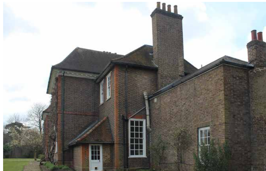
3.8 The northern extensions on the east side (looking south)
