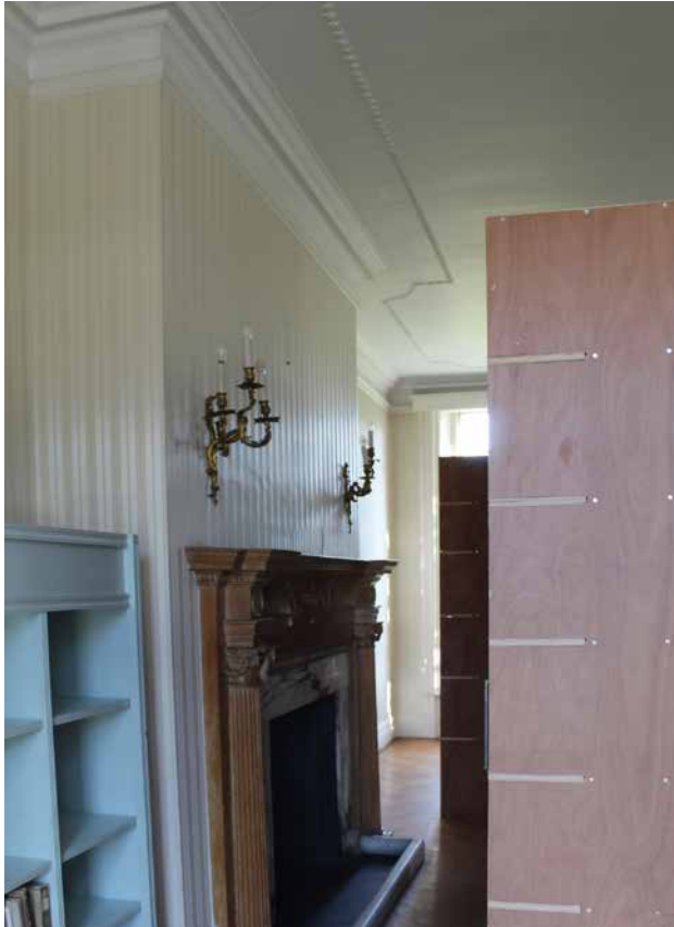
3.28 The southern room at ground floor level (G7) looking east
