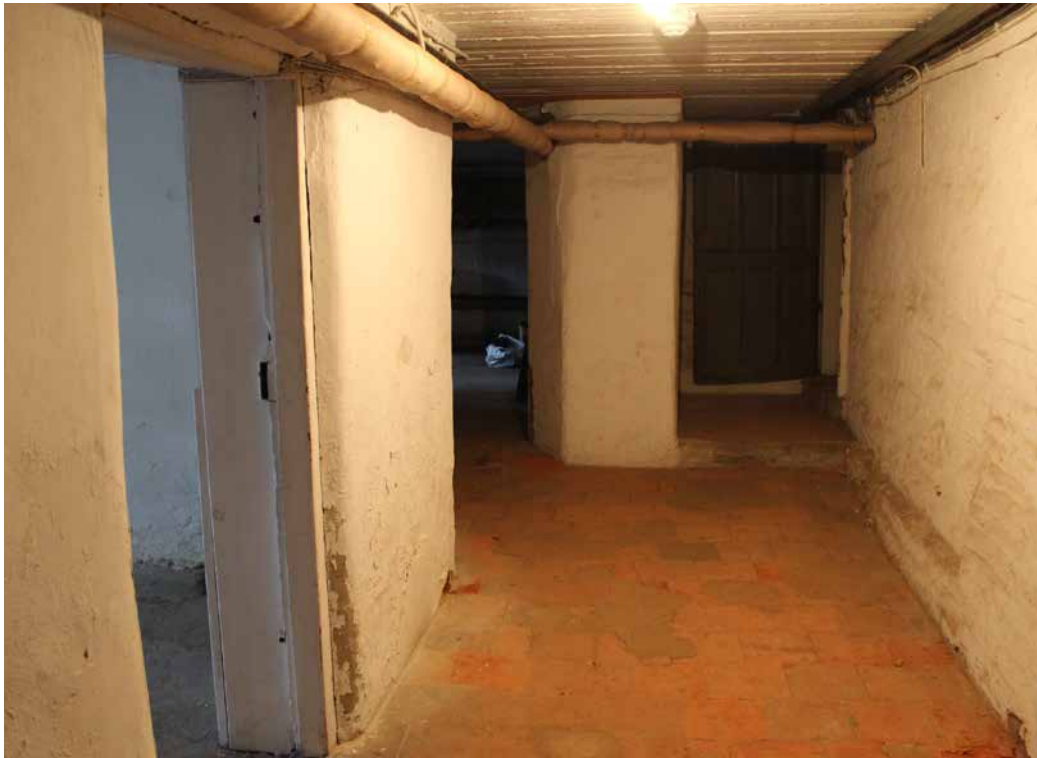
3.11 The basement corridor (B4) looking south
