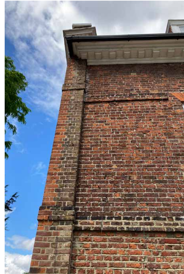
3.4 The west facade (left) projects beyond the face of the earlier south facade (right)
