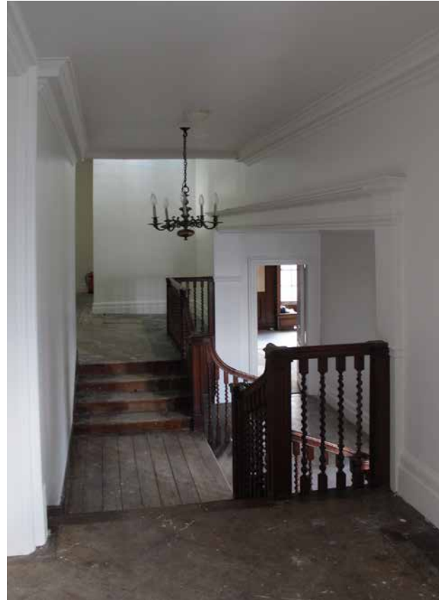
3.29 The Edwardian corridor and stairs at first floor level looking south
