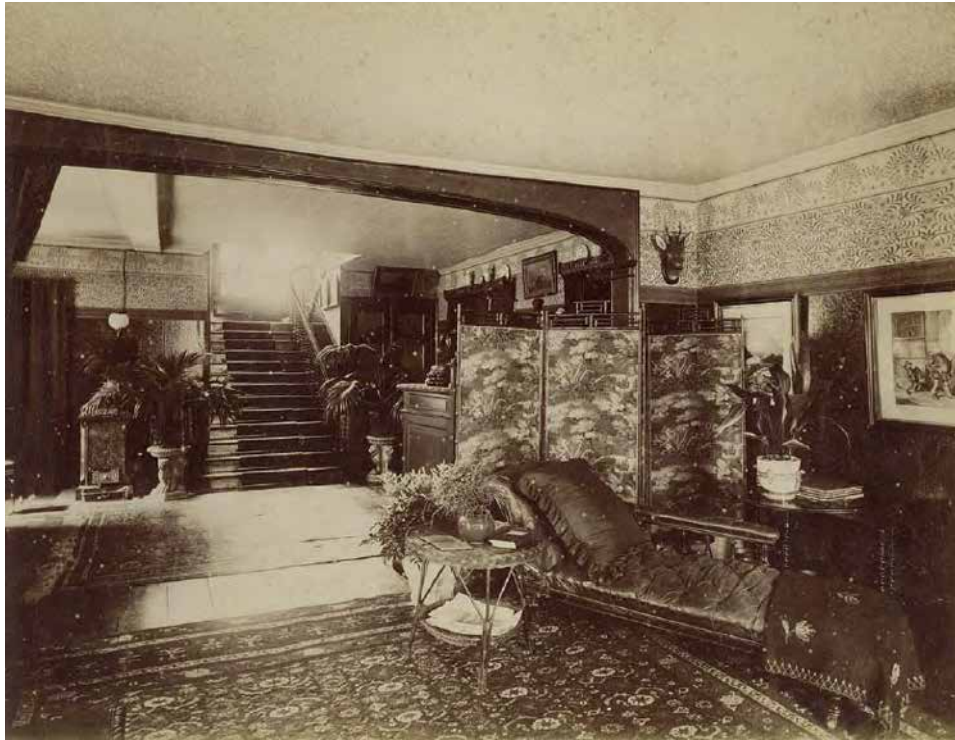
5.1 Room G4 Looking North (OA)
