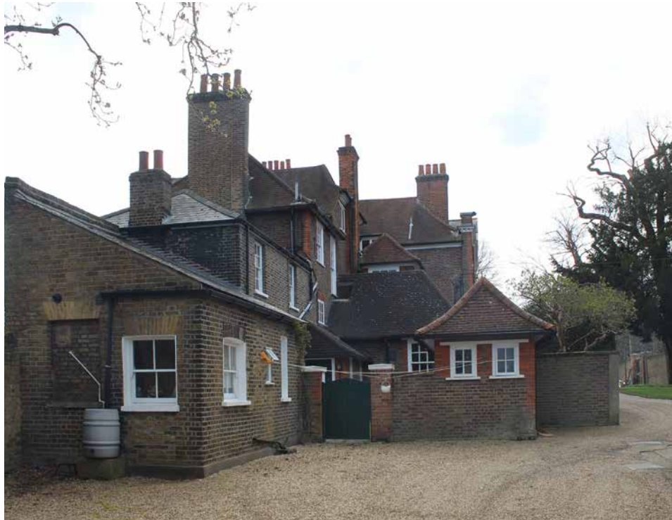
3.5 The extensions north of the original house (west side, looking south)
