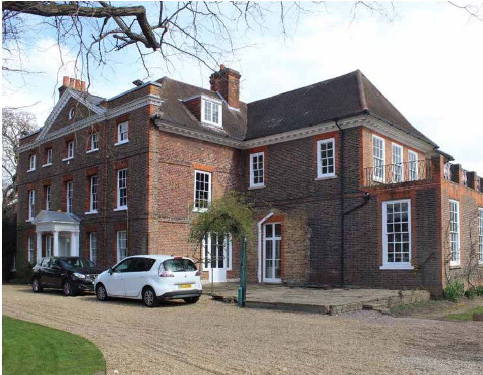
3.3 The west (front) facade from the southwest with the Edwardian extension (right)
