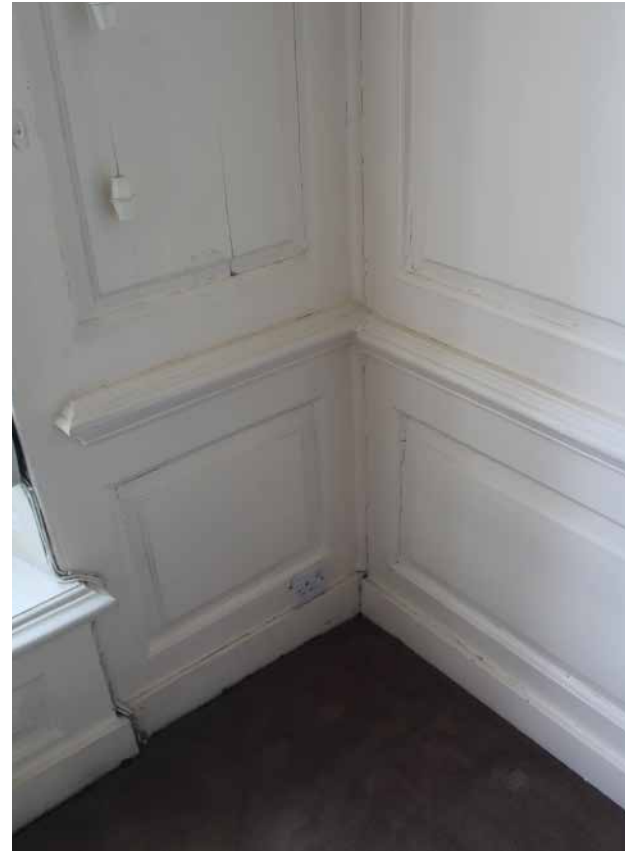
3.19 The northeast room (G1). Junction of later south partition wall with 18C east wall
