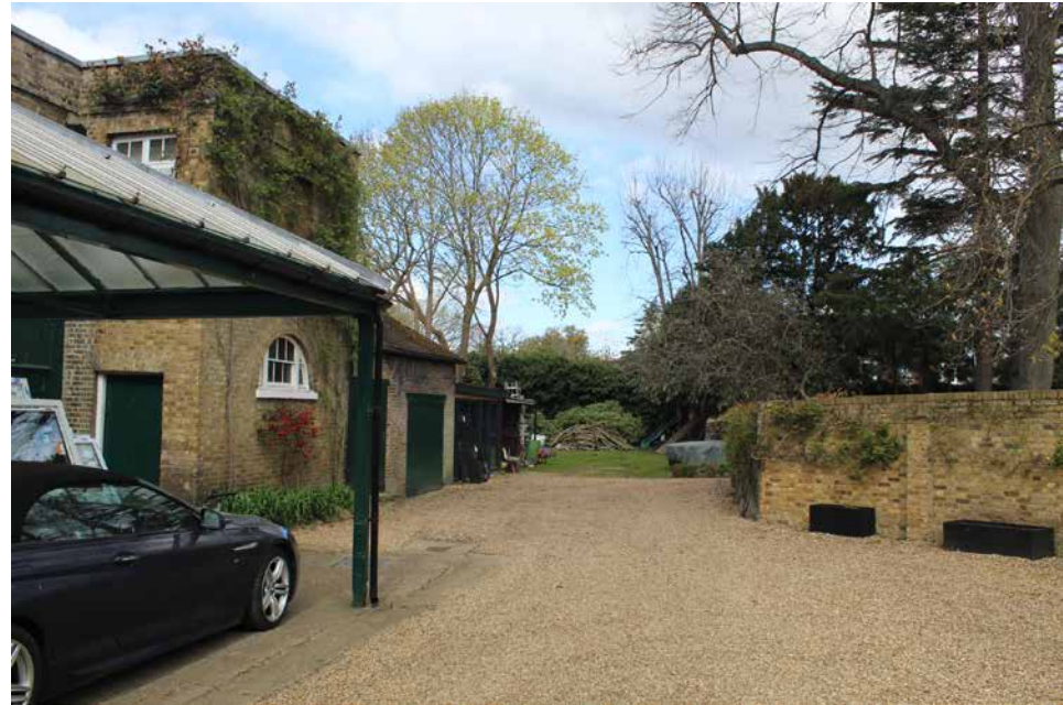
5.4 View northwards showing the north end of the garages, where the approved extension will be (left)
