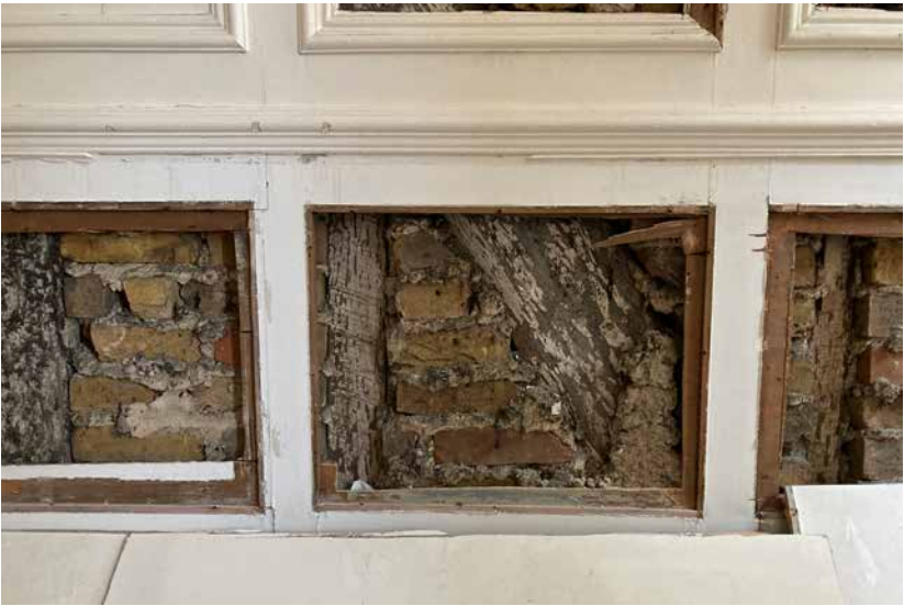
3.22 Close up of the timber framing with brick infill (F2)
