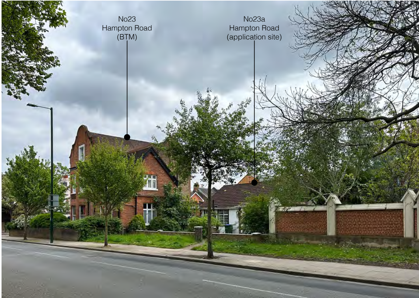
View (looking south east) along Hampton Road towards No23a application site and neighbour, No23 (BTM).
