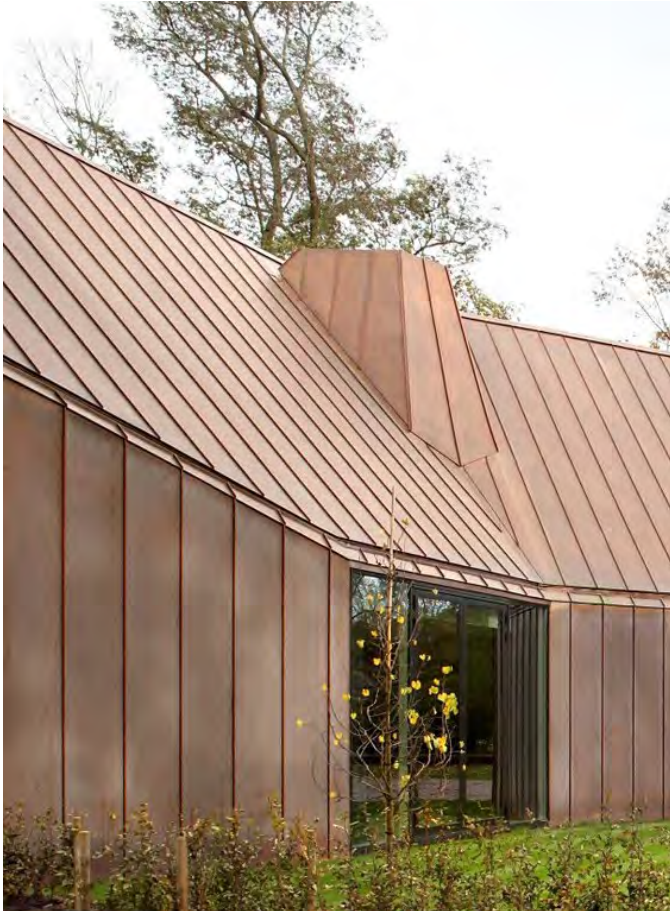
Copper cladding; responding to the red tonality of the neighbouring buildings.
