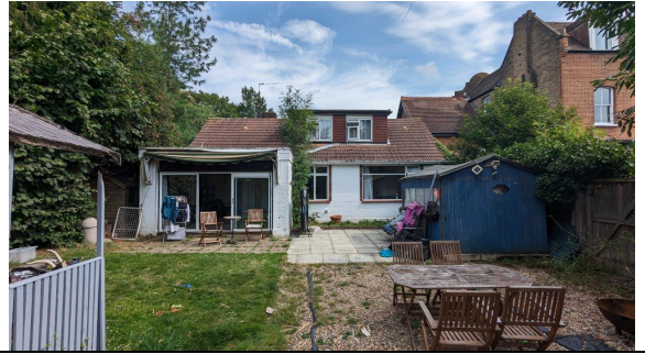
Photo 2. The northern elevation and garden shed 1. No external potential roost features for bats were found.
