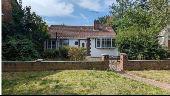
Photo 1. The northern elevation. No external potential roost features for bats were found.
