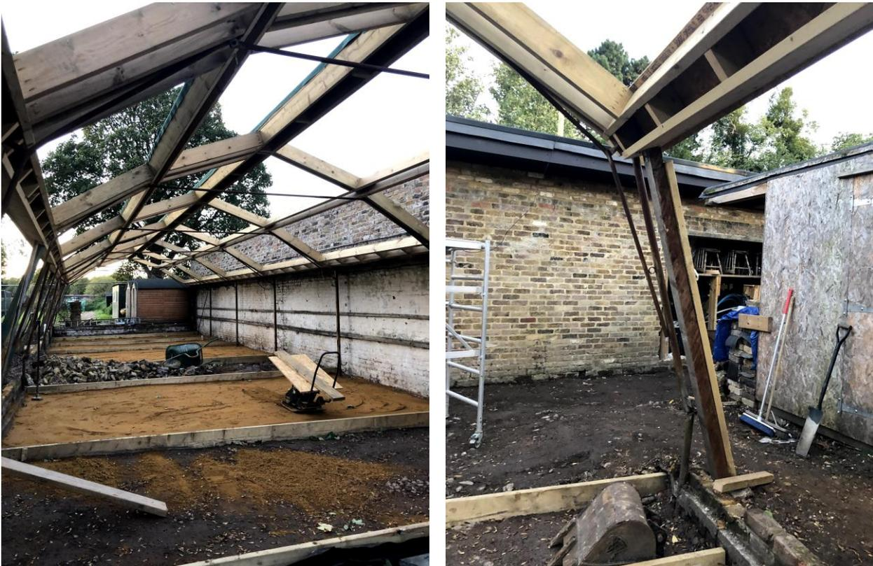
Figure 29 – Building D in construction showing the metal pole frame of the former glasshouse that was reused
