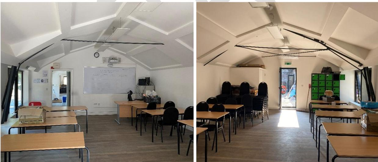
Figure 30 - Building D interior with salvaged metal pole structure from former glasshouse
