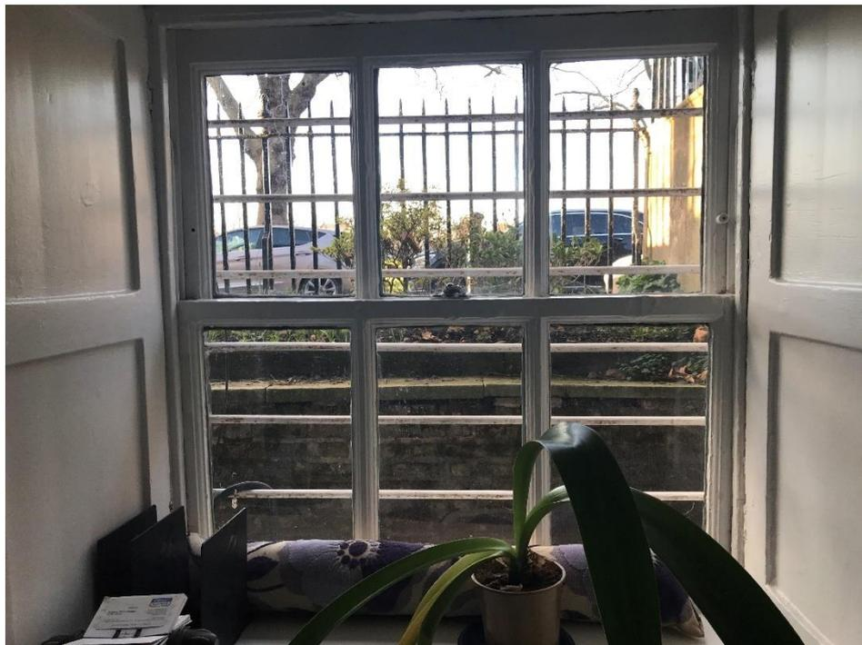
*Figure 7: Sash windows to the front lower ground floor opening have very thick glazing bars with traditional mouldings typical of the first decades of the 18<sup>th</sup> century*
