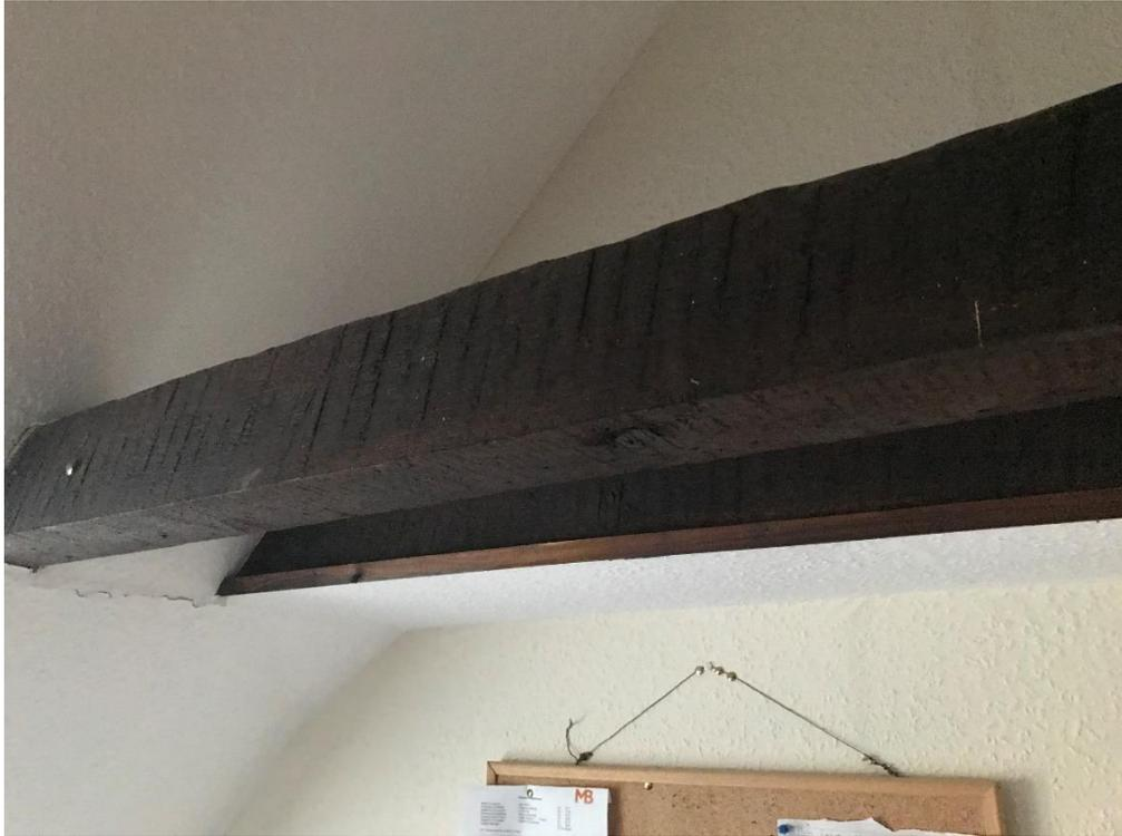
*Figure 33: Evidence of hand sawn timbers to ties of the M-shaped roof at attic level. The timbers were previously underdrawn by a lath and plaster ceiling with the rooms originally serving as quarters for domestic staff.*
