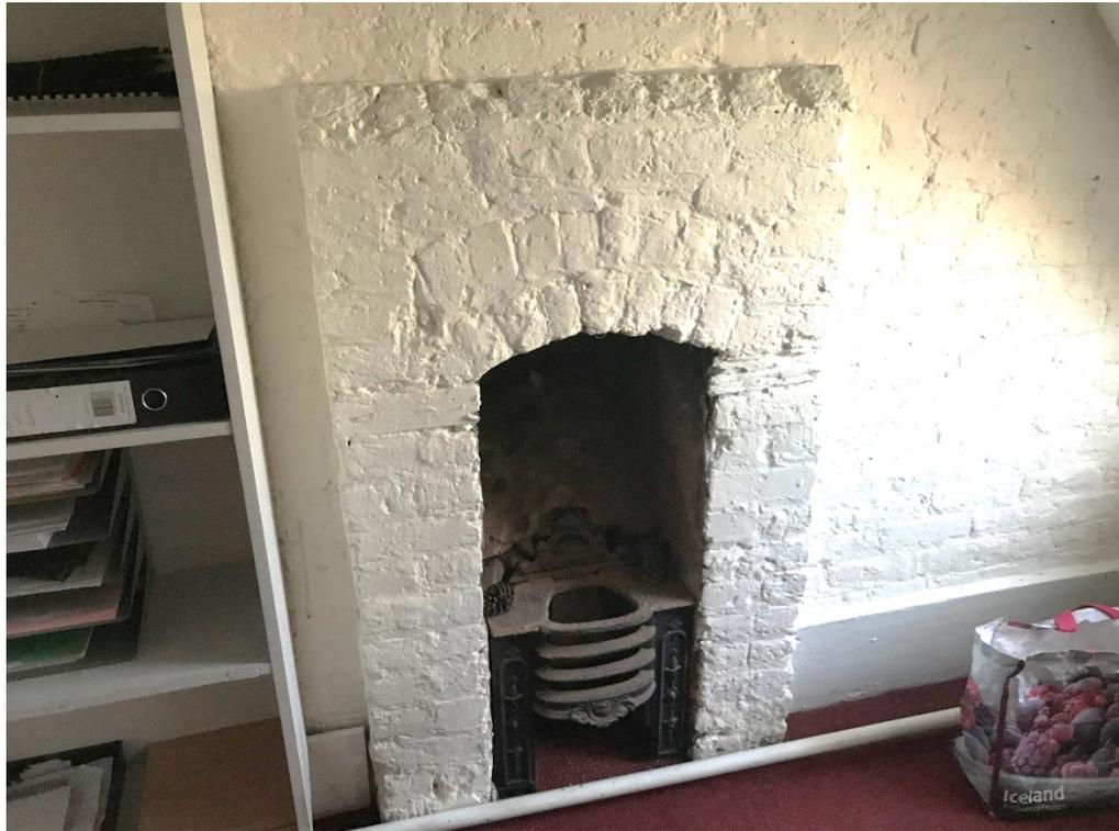
*Figure 29: Attic room fireplace with original coal grate*
