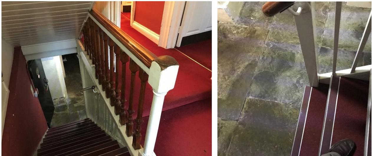
*Figure 30: Basement stair with original riven York stone floor retained throughout*
