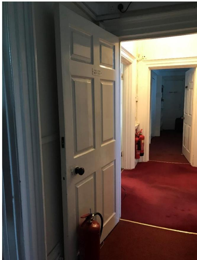
*Figure 22: Raised and fielded panelled doors at first floor level*
