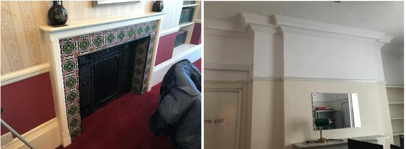
Figure 25: Moulded skirting, dado detail (left - ground floor) and picture rail / cornicing (right - first floor) typically found throughout the house
