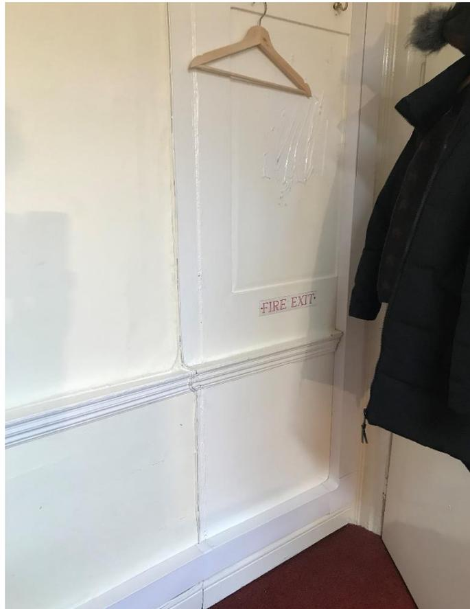
*Figure 32: Jib door at second floor level*
