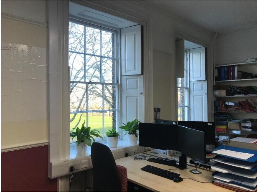
*Figure 31: Typical late 18<sup>th</sup> century sash window detail to first floor left hand reception room. A high proportion of mouth blown cylinder / crown glass appears to survive within these historic window frames.*
