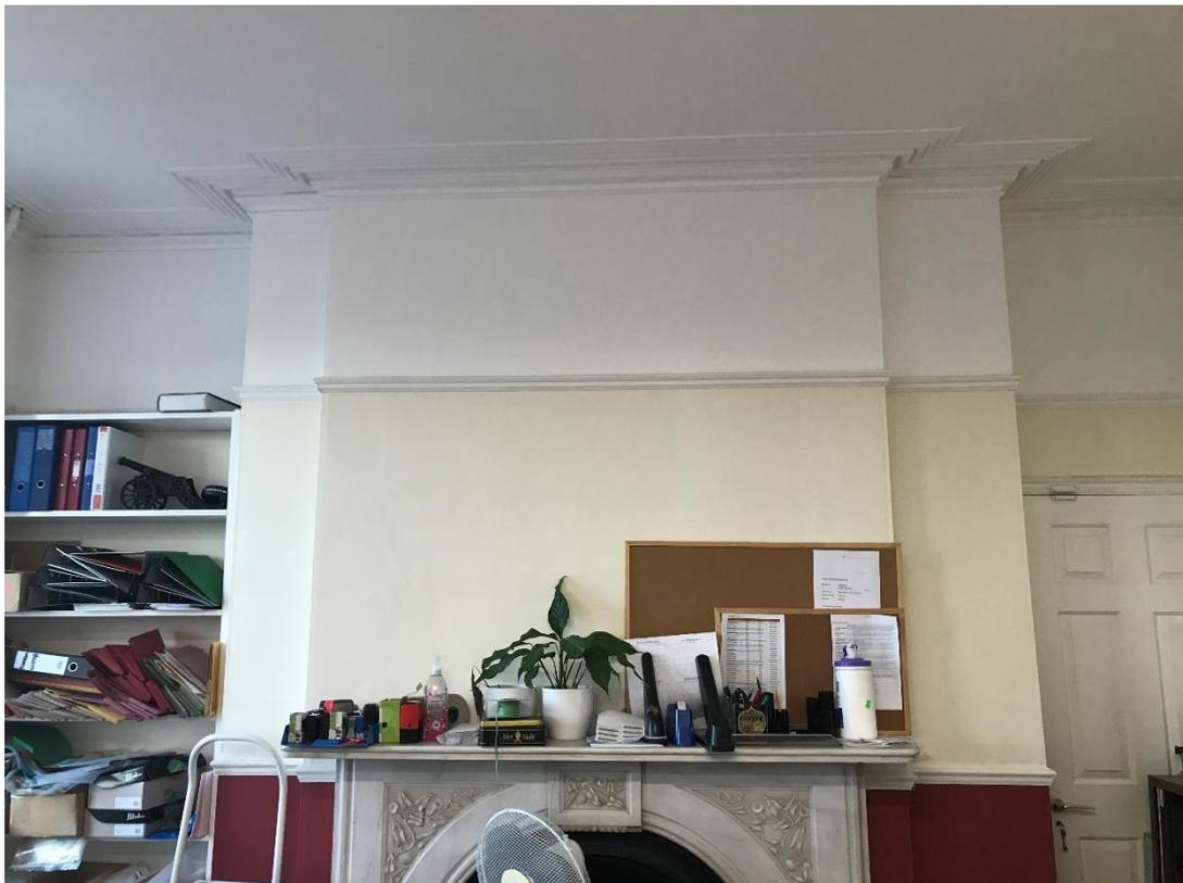
Figure 26: Good quality cornicing with cabled moulding at first floor level (left hand reception room)
