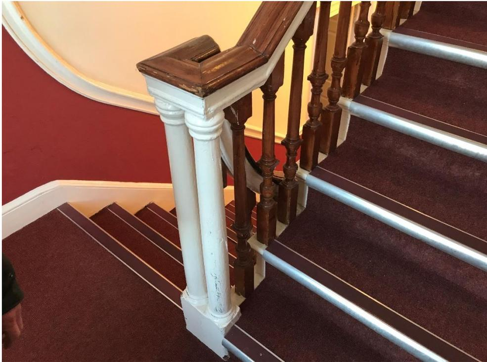
*Figure 9: Staircase newel post detail of paired Tuscan columns*
