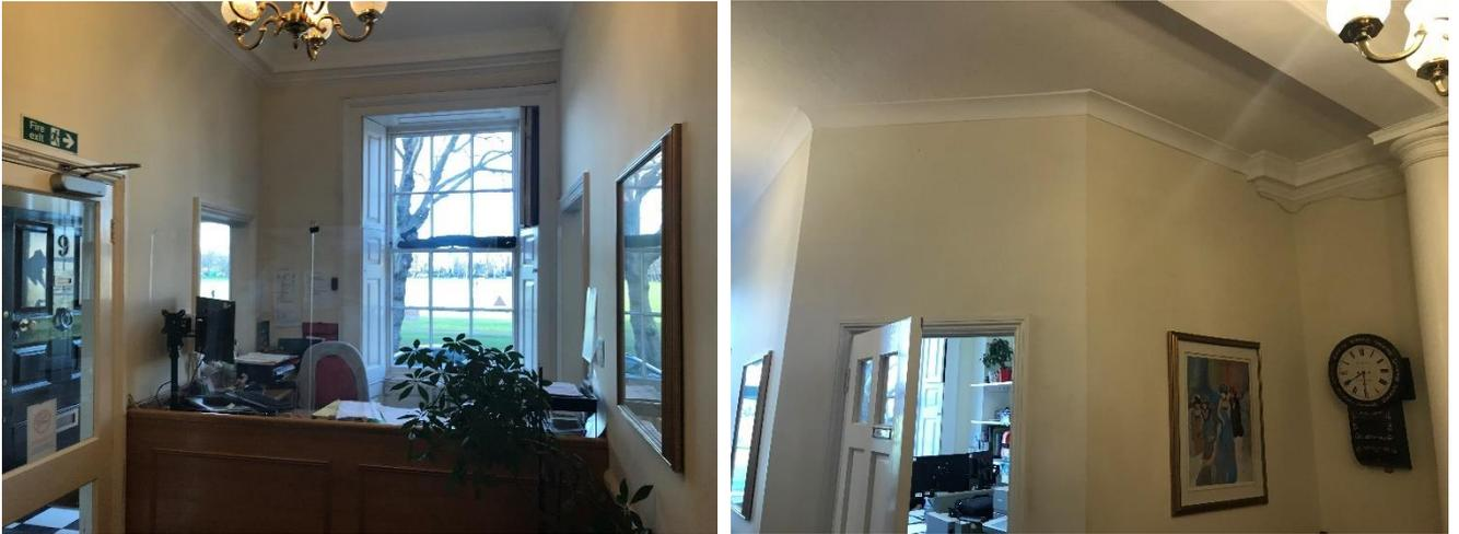
*Figure 35: Late 20<sup>th</sup> century partition to ground floor left hand reception room installed to create a receptionist's office and front of house reception desk.*
