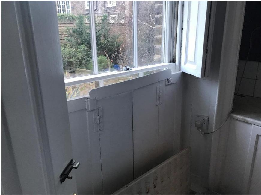
*Figure 21: Typical window shuttering to a rear window. Shutters remain to almost all the windows in the house*
