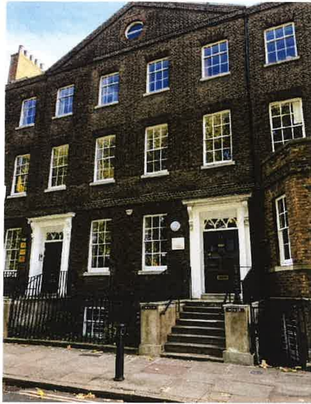
Front of building.
