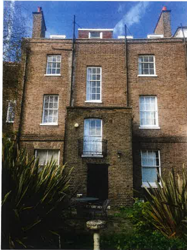
Rear of building.
