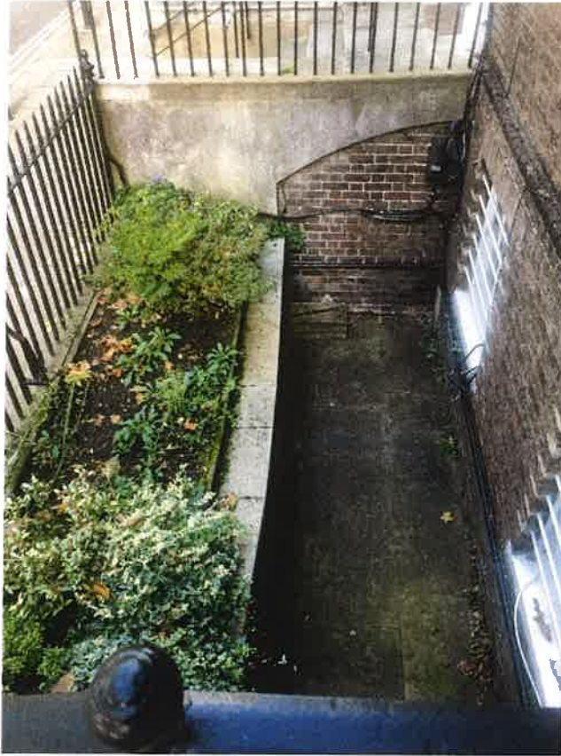
Lower ground floor at front of building.
