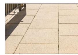
Goundfloor Patios Paving slabs: Mayfield supplied by Tobermore or similar equivalent; Colour: sandstone; non-slip textured slabs installed in accordance with the manufacturer's instructions
