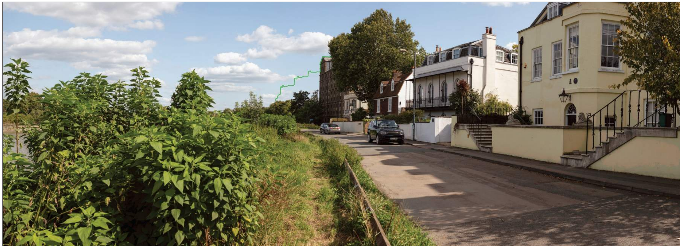
Viewpoint 2: Proposed view from Thames Bank adjacent to the University Boat Race marker looking south east towards the Site.
