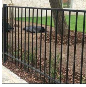
Example 10. Road Frontage boundaries: Flat top railings 1200mm high; supplied by Alpha Rail or similar equivalent
