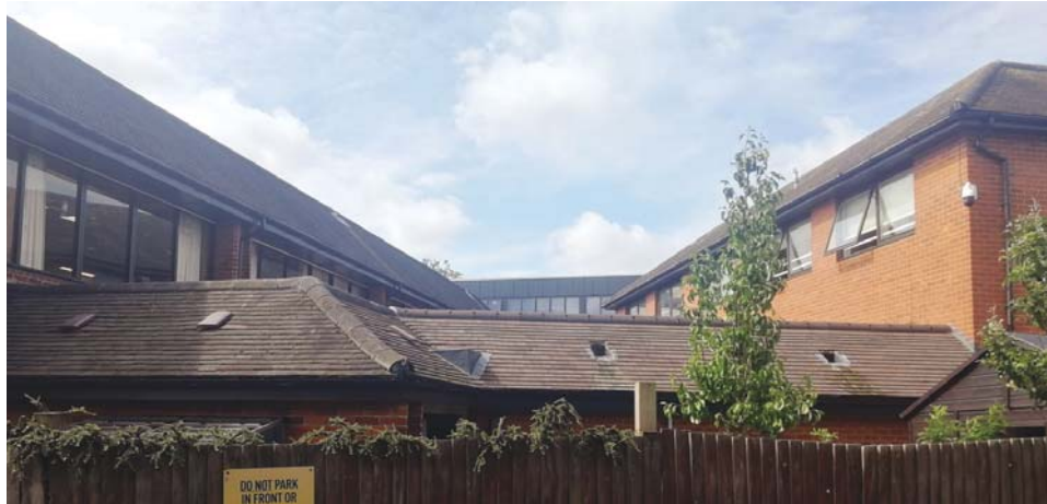
Existing view from Grotto Road, looking south
