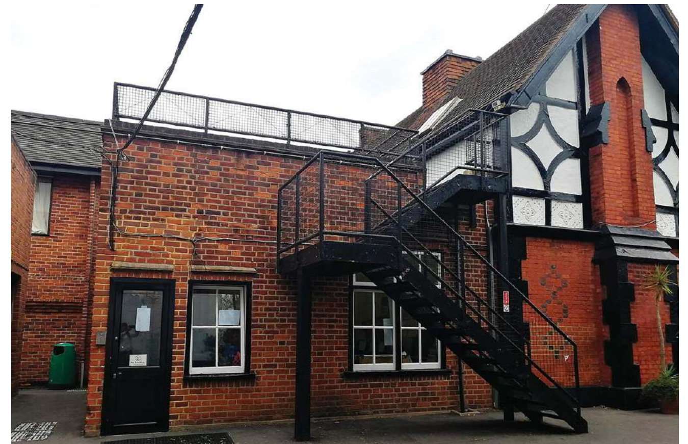
Photo of the Lodge and extension taken within the site (looking north-east), 02.08.22
