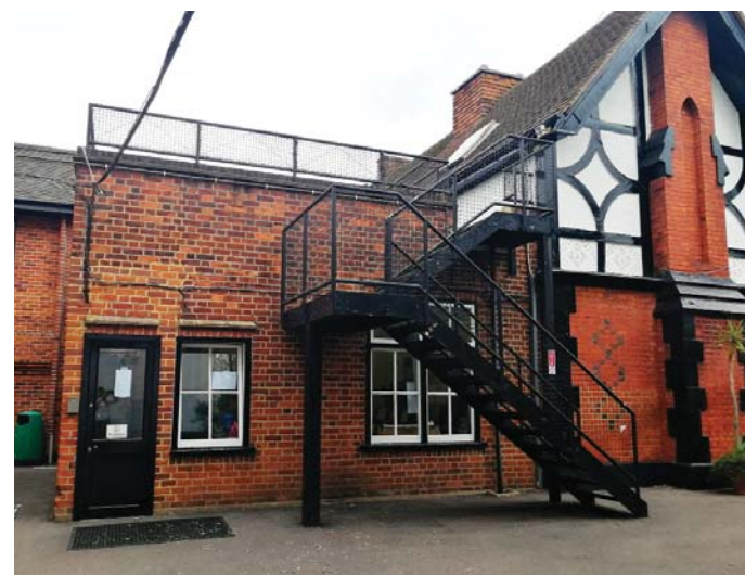
The 20th century extension at the rear of the Lodge
