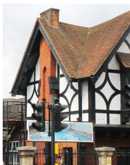
The Lodge with red brickwork
