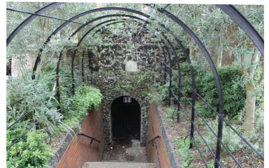
Steps and entrance to the tunnel to Pope's Grotto
