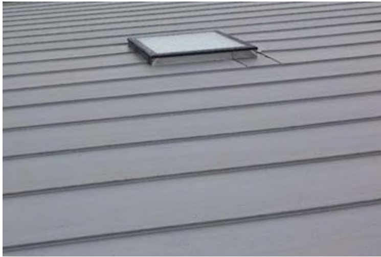
Shallow pitch standing seam zinc roof with rooflight
