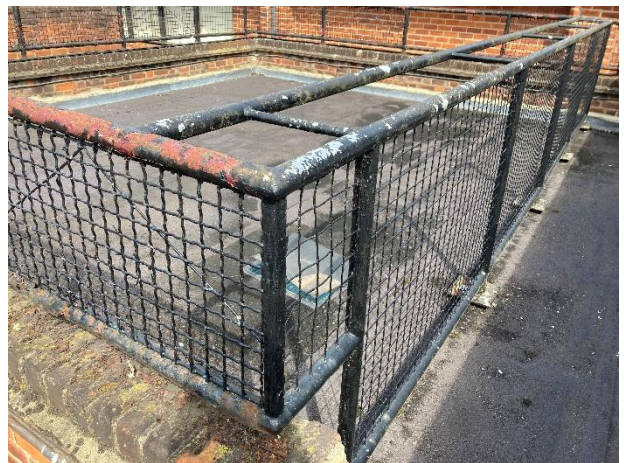
Photo 5, "Roof of Building B2"
