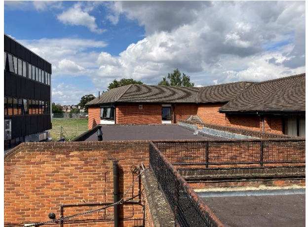
Photo 2, "Roof of B1"
