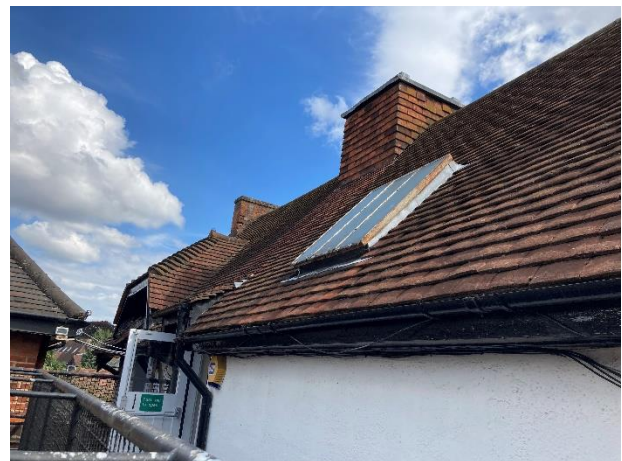
Photo 8, "Roof of the Lodge"
