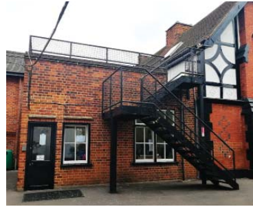
Existing extension and fire escape to the Lodge, to be removed.
