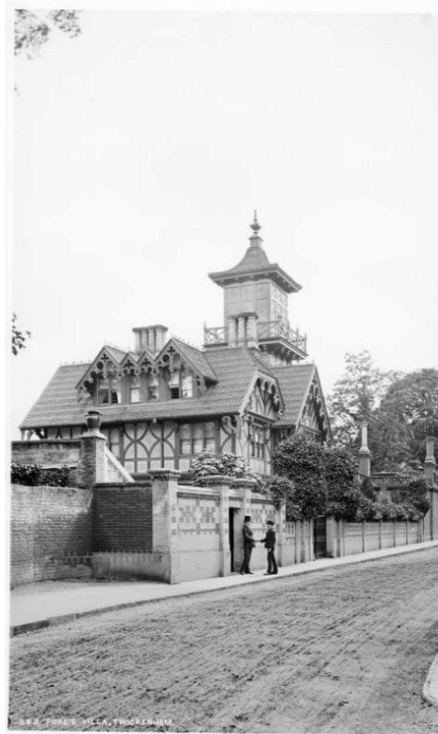
Figure 7: Exterior view of Pope's Villa approximately at the time when St Catherine's Convent first occupied the building (Source: Historic England Archive)
