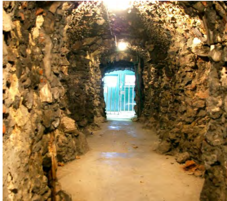
Figure 30: The tunnel looking towards the river Thames. The view to the river is blocked by a building. (Source: Pope's Grotto Preservation Trust)
