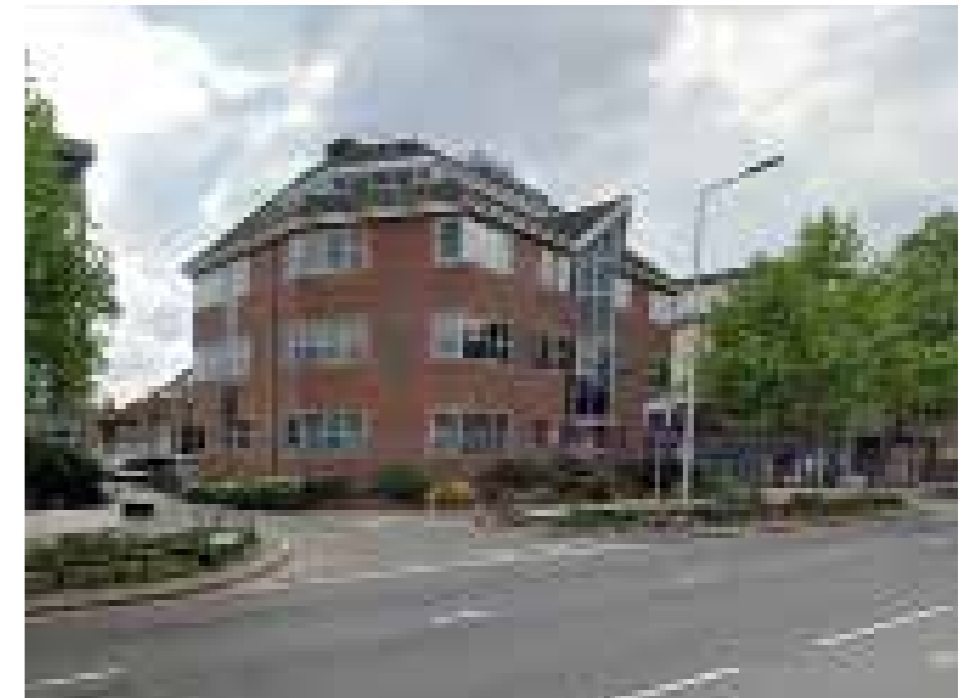
Existing street view
