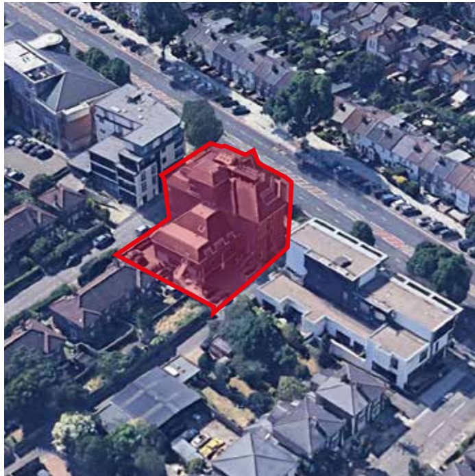
Aerial view from south east
