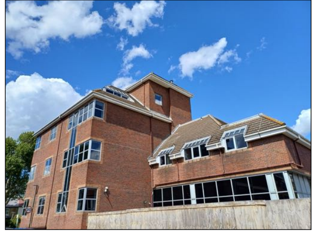
Image 5: A view of the south and west elevations of the building.
