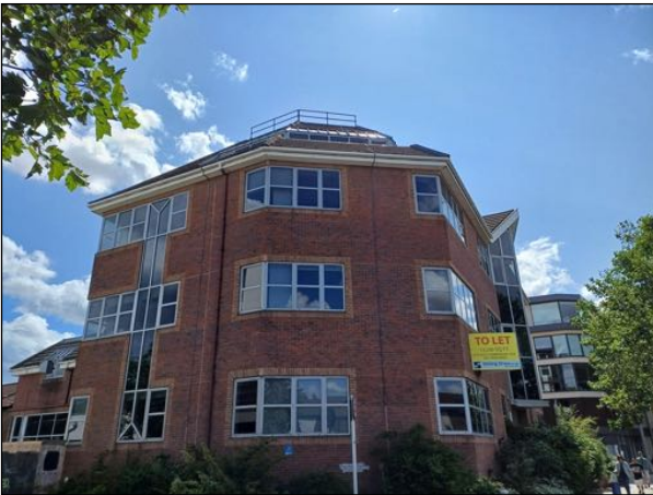
Image 6: A view of the east elevation of the building.
