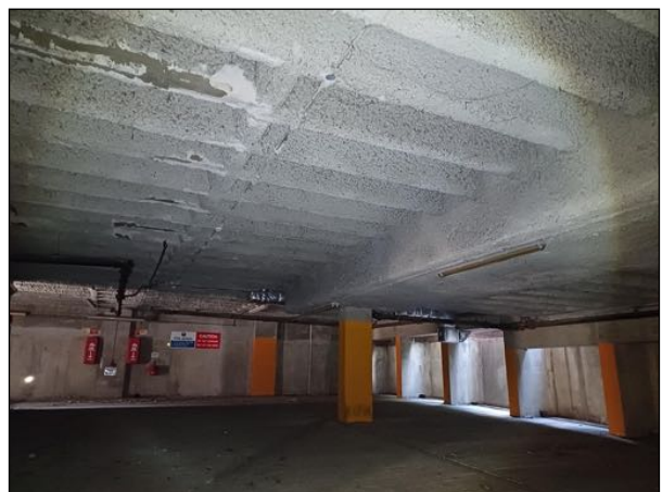
Image 15: View of the basement car park.
