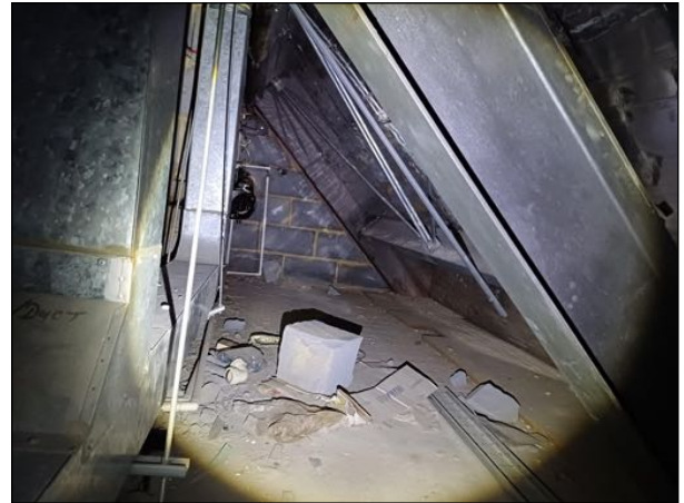
Image 11: There is a small crawl space on the second floor.
