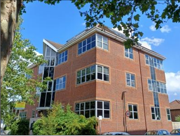
Image 4: A view of the northwest corner of the building.
