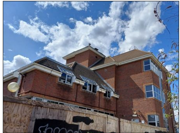
Image 7: A view of the south and east elevations of the building.
