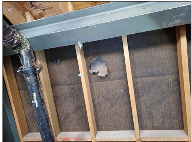
Image 13: One of the lift shafts present is open from the top floor void space but has no roosting opportunities.
