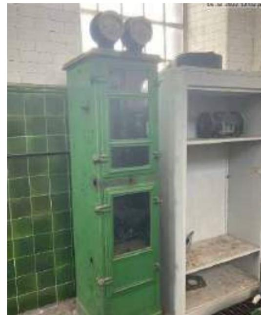
Harland control cabinet for electric centrifugal pump
