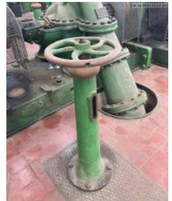
Valve Control standard for centrifugal pump
