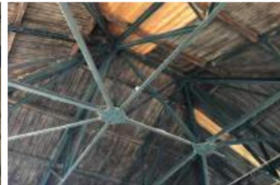
Intricate wrought iron truss work holds up the timber and slate roofs
