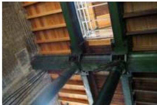
Tuscan order steel columns hold up the second floor's large steel beams in The Beam, Karslake
