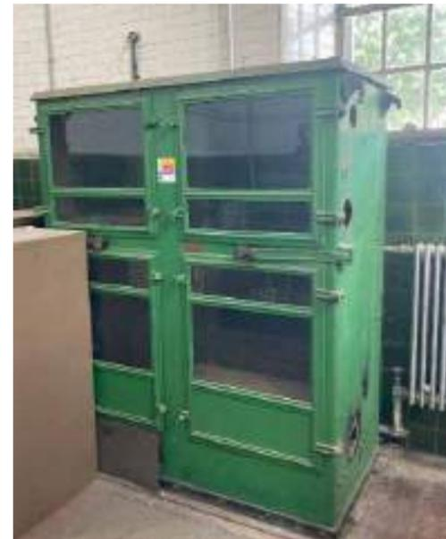
Harland control cabinet for electric centrifugal pump
