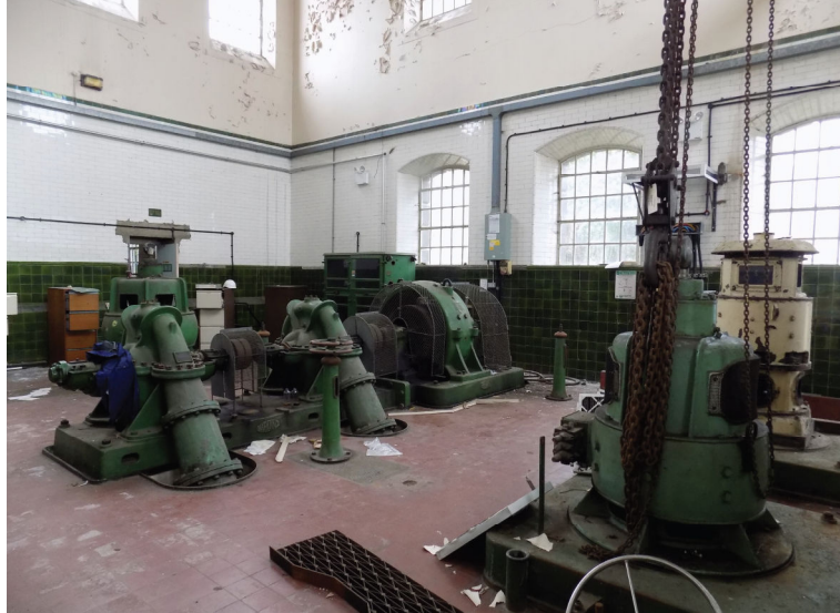
Figure 1 – Wall tiles / Floor tiles
