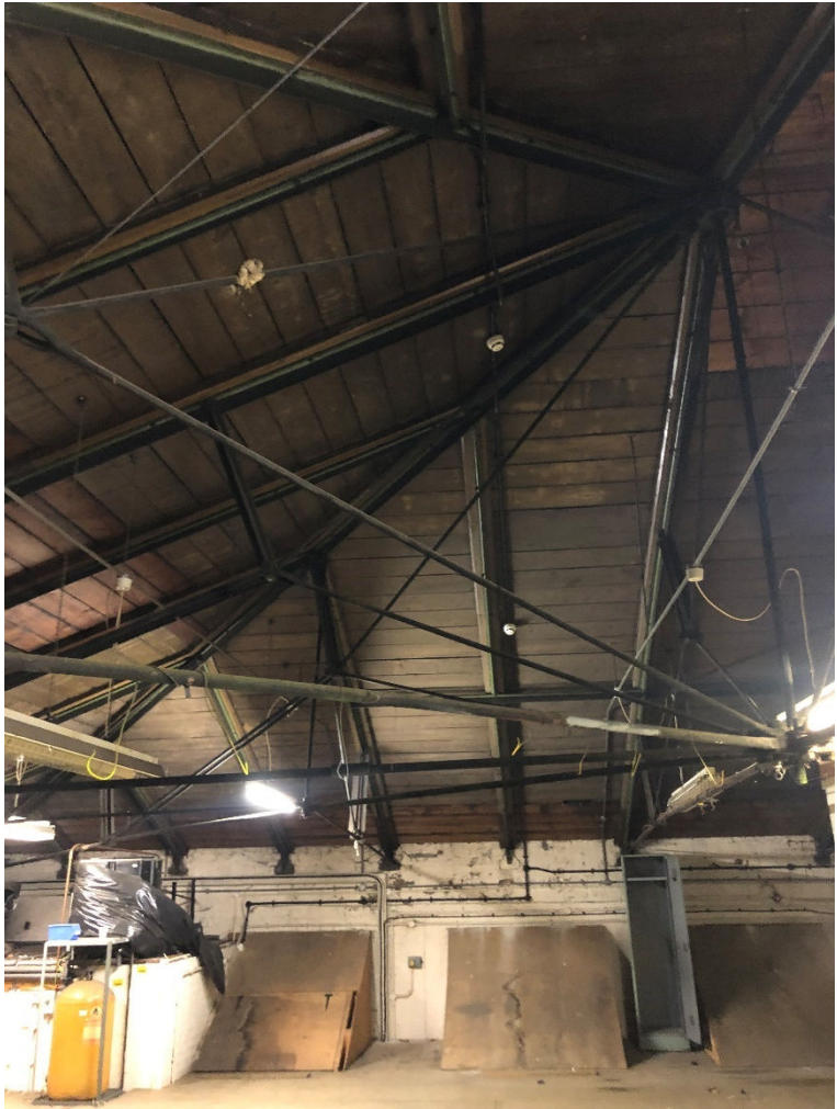
Reference: Figure 18 – Primary wrought iron roof structure
