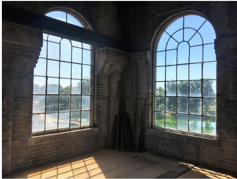
Figure 15 – Cast Iron windows
